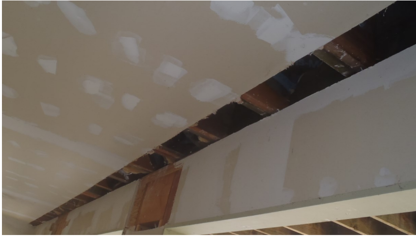
Photo: The contractor removed part of the ceiling to access the floor framing and install shear transfer ties.
