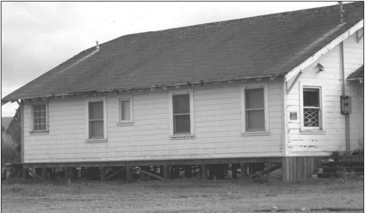
Fig.6. 2 House with Braced Posts along Perimeter
