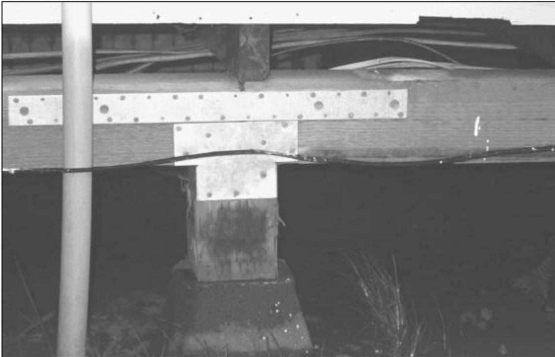
Fig.6. 5 New Metal Strap Reinforcement
