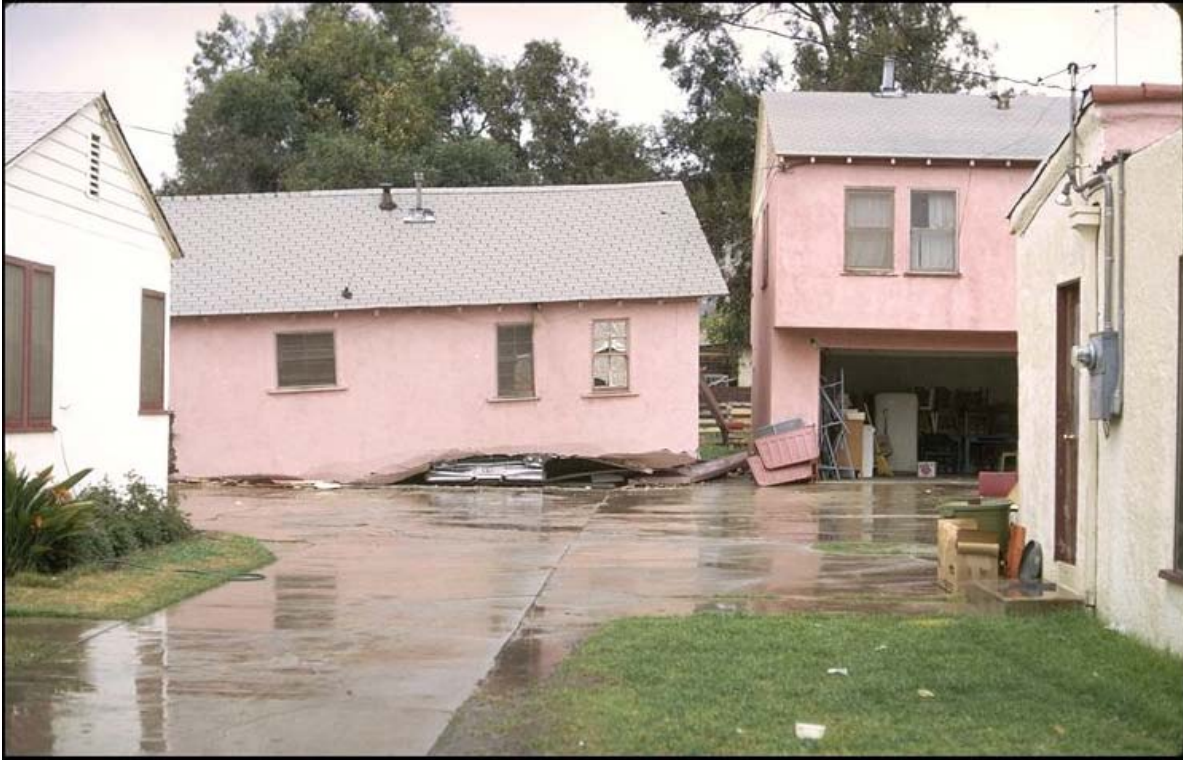
The building on the left used to be two stories. This collapse was caused by overturning of tall narrow shear walls that could not resist the earthquake forces generated by the heavy living area above a garage
