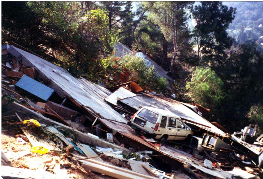
EARTHQUAKE DAMAGE TO HILLSIDE HOME IN NORTHRIDGE EARTHQUAKE
