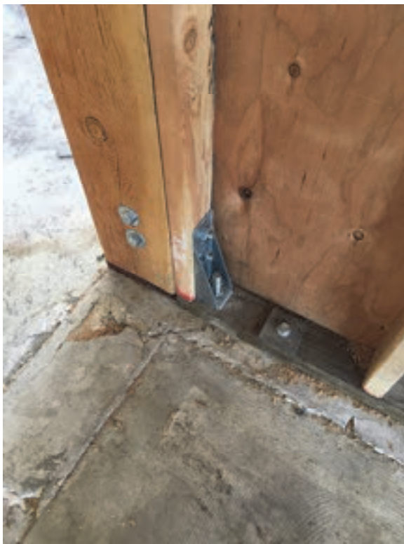
Figure 2-31 Tie-down at end of wood structural panel shear wall (photo credit: E. Mikailian).
