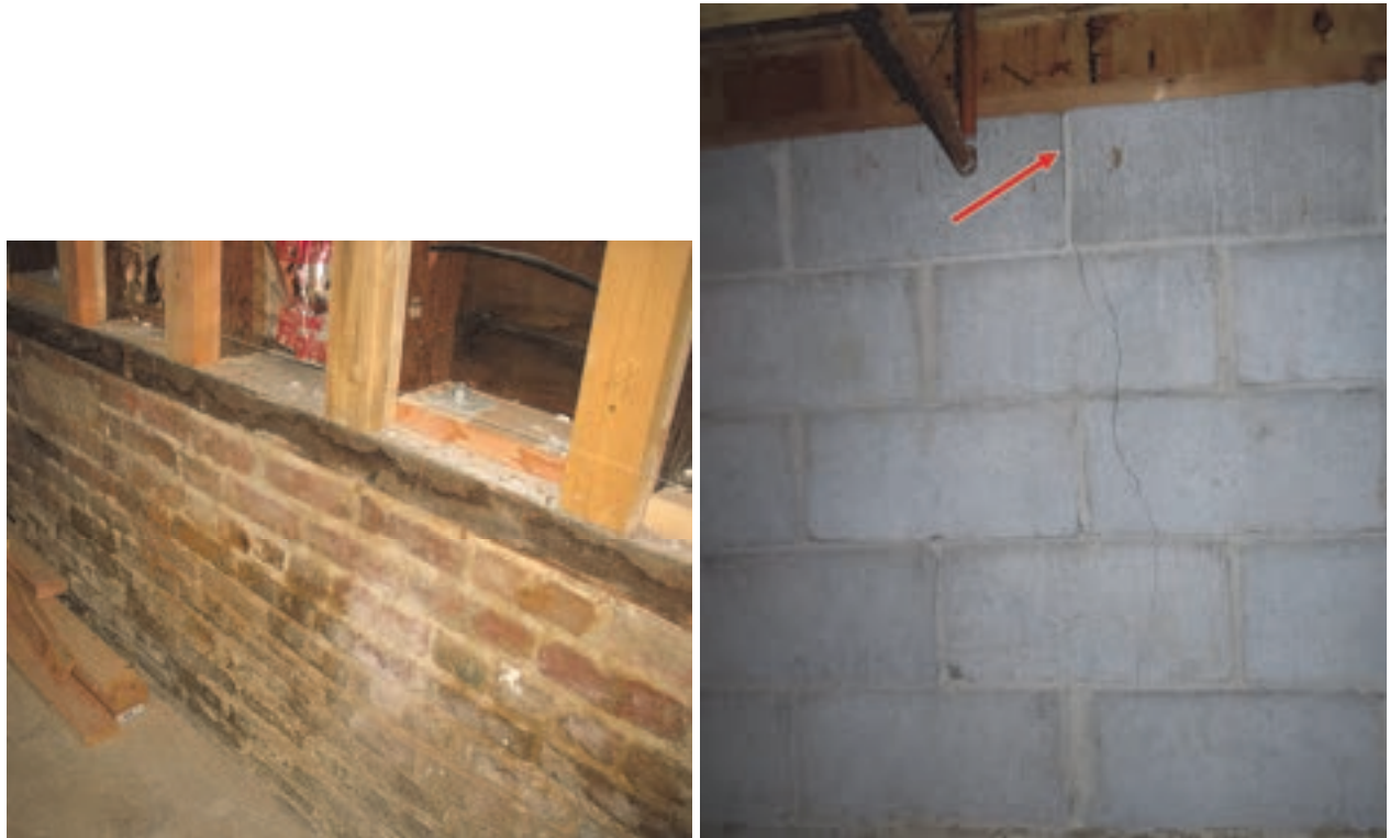
Figure 2-16 Typical brick masonry (left) and CMU (right) basement wall configurations, where cracking in the right photo was caused by the 2018 Anchorage, Alaska earthquake (photo credits: D. Bonowitz, left, and Z. Stutts, right).
