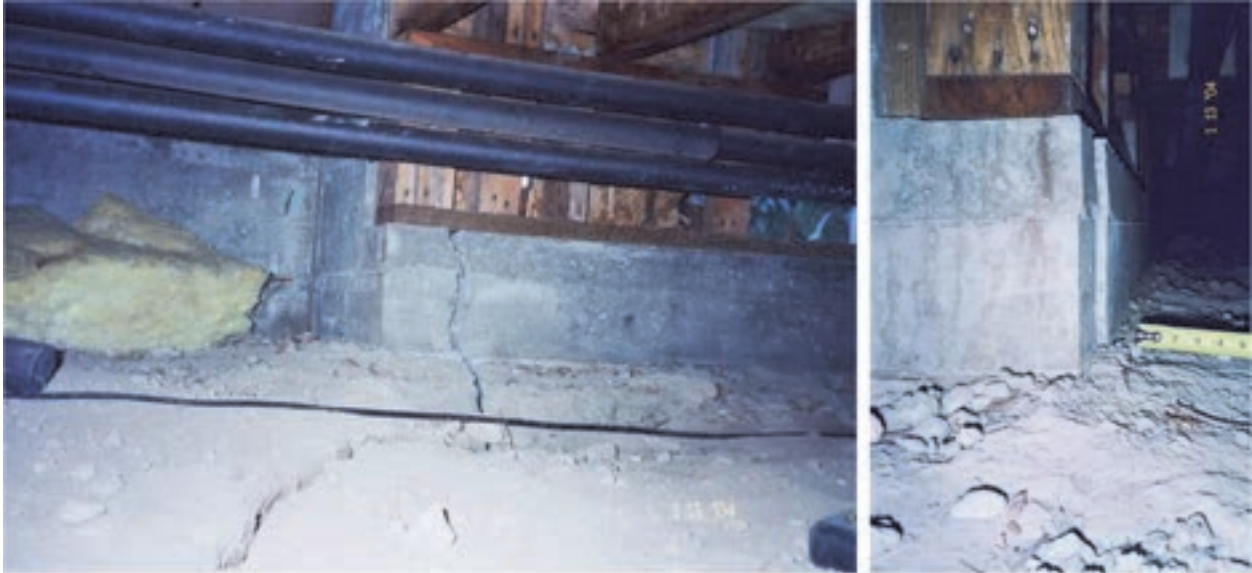
Figure 6-11 Foundation and ground cracking following the 2003 San Simeon, California earthquake, where the photo on the right shows the offset present across foundation crack (photo credits: Exponent).
