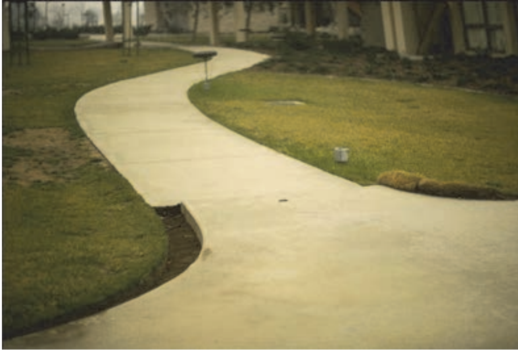
Figure 6-8 Offset sidewalk from the 1971 San Fernando, California earthquake (photo credit: NISEE).
