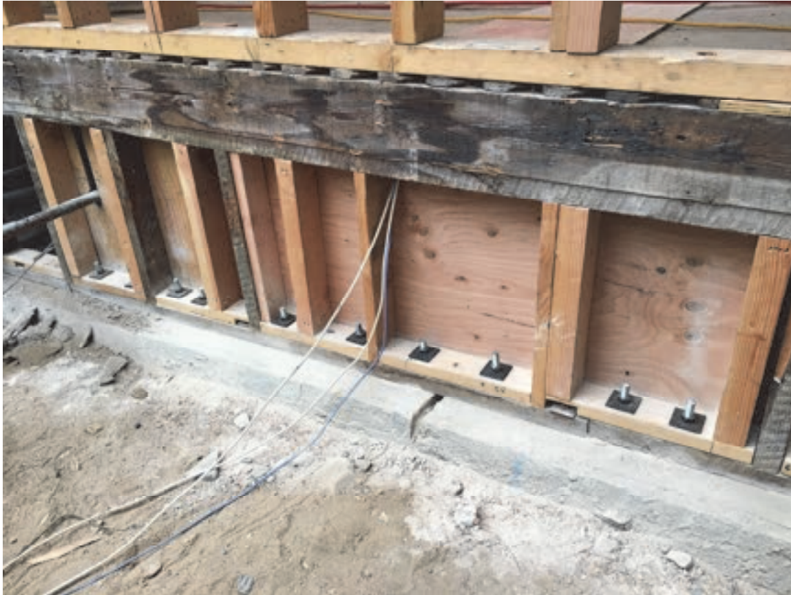
Figure 2-19 Steel post-installed anchor bolts associated with modifications to a house. These are adhesive anchors attached to an existing concrete foundation (photo credit: E. Mikailian).
