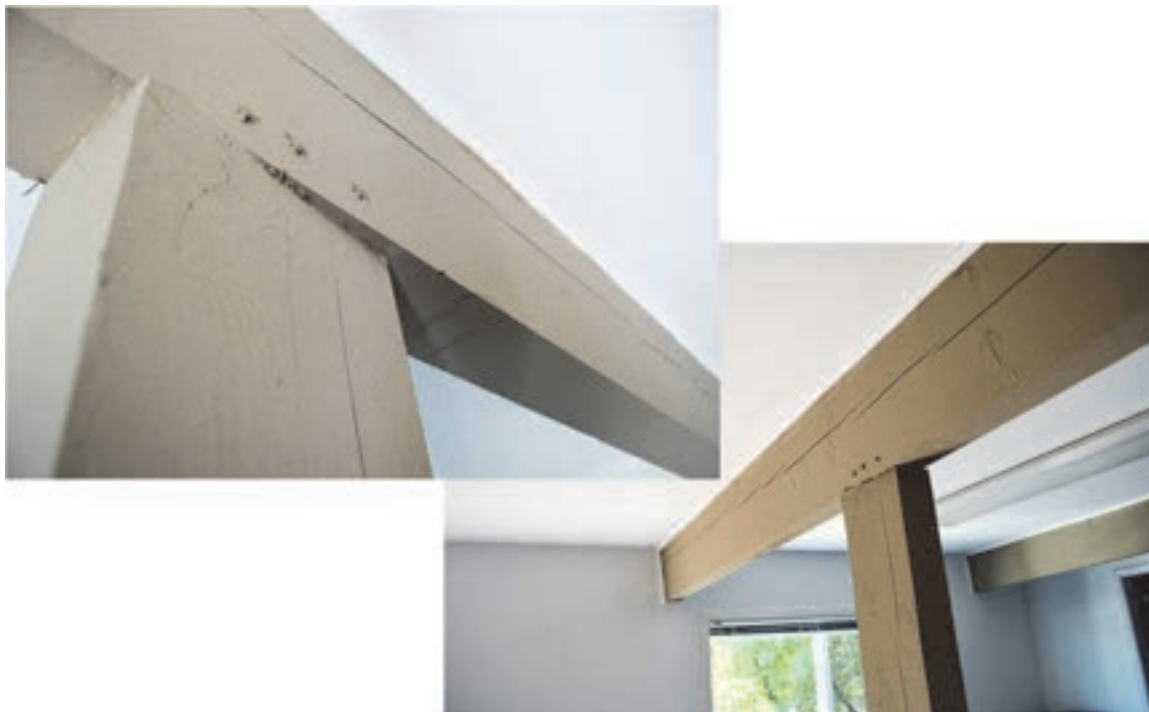
Figure 2-32 Gravity-load-carrying post supporting a beam. The two members, which are toe-nailed together, are misaligned, but lack of an unpainted surface indicates no recent relative movement (photo credit: Exponent).
