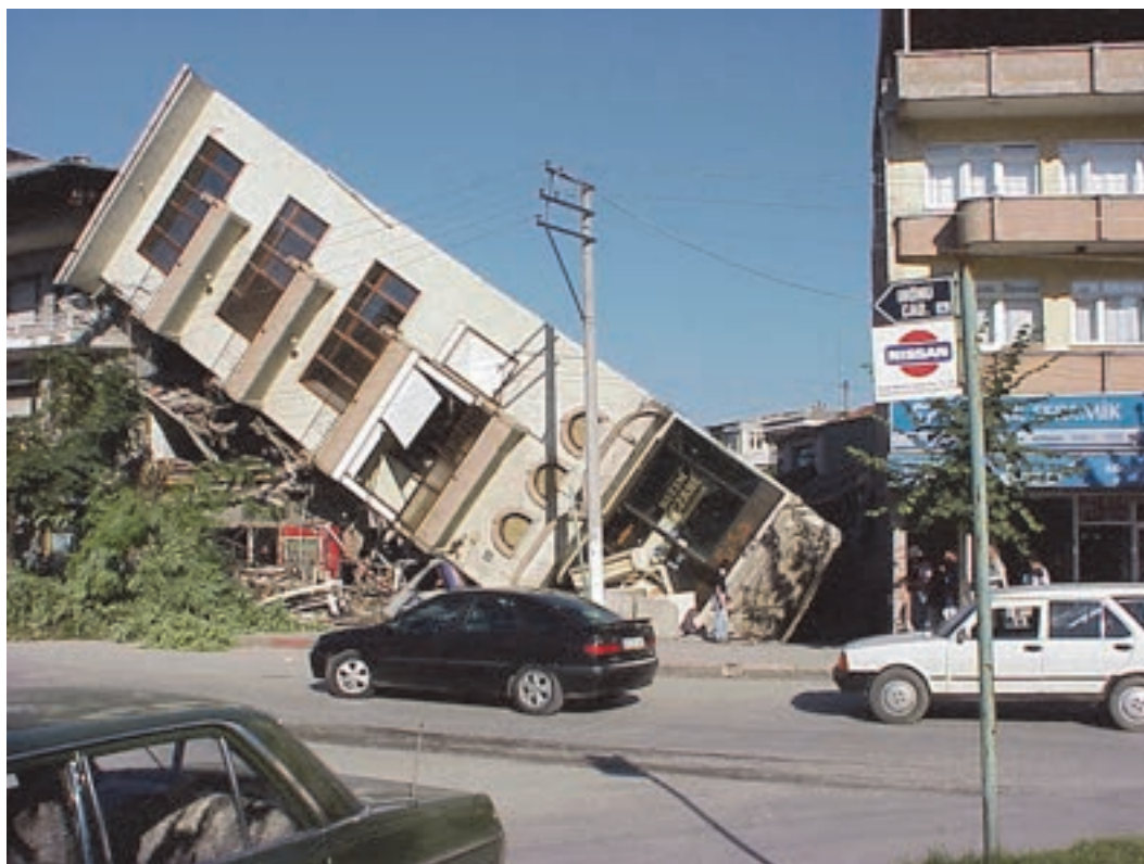
Figure 5-13 Foundation bearing failure of shallow foundation in Adapazari from the 1999 Kocaeli, Turkey earthquake (photo credit: J. P. Stewart).
