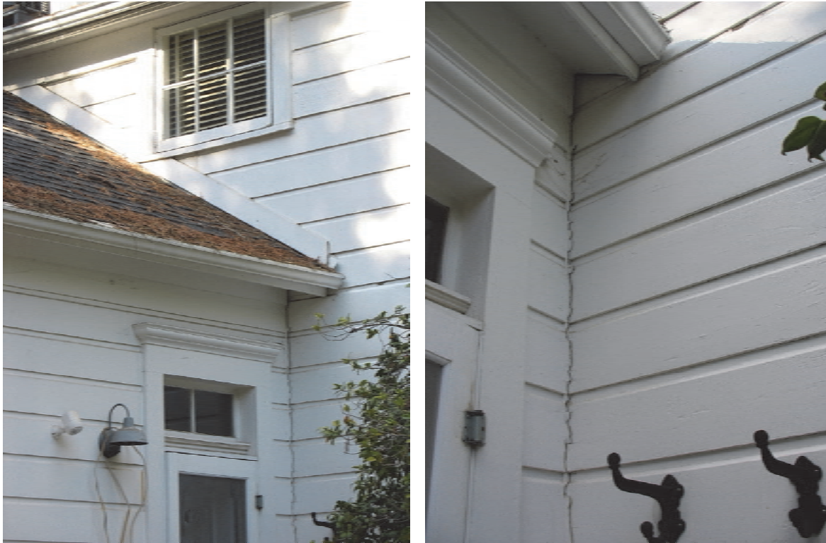
Figure 2-9 Left: Adjoining wings of a house create a framing discontinuity. Right: Separation of wood siding at intersection of adjoining wings caused by the 2014 South Napa, California earthquake. The separation was not structurally significant because there was no continuous framing or structural connection between the wings (photo credit: D. Bonowitz).
