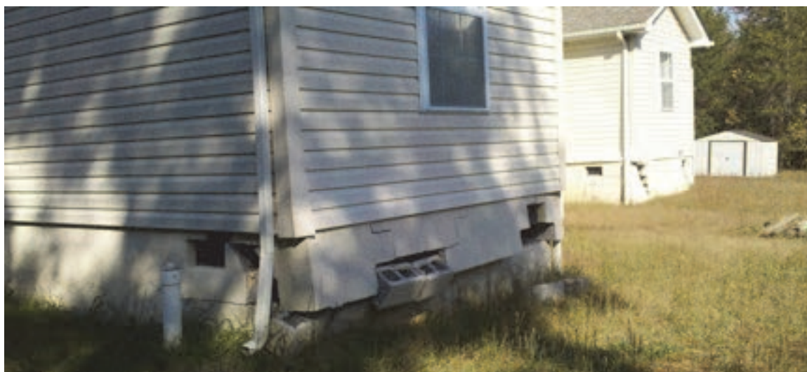
Figure 2-12 Damage of unreinforced, ungrouted masonry stemwalls caused by the 2011 Virginia earthquake (photo credit: M. Mahoney).
