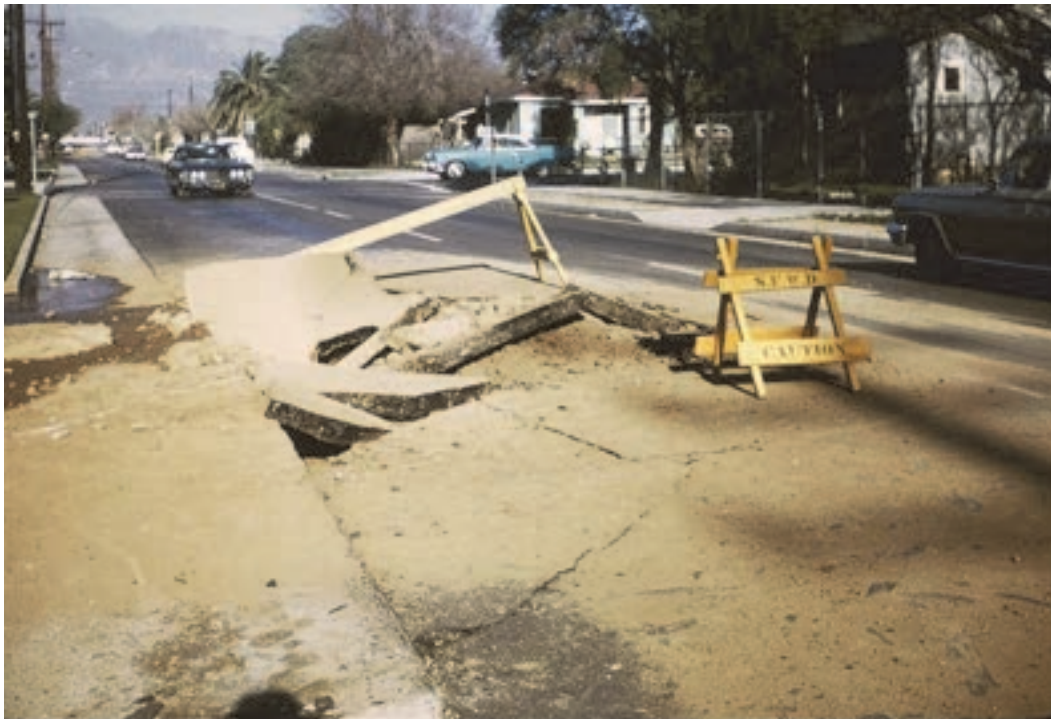
Figure 6-2 Pipe failures and resulting pavement distress and settlement from the 1971 San Fernando, California earthquake (photo credit: NISEE).
