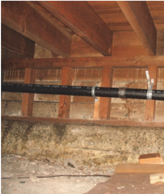
Figure 2-17 Sill plate below cripple wall framing of older house with steel post-installed anchor bolts attaching the sill plate to the foundation (photo credit: D. Bonowitz).
