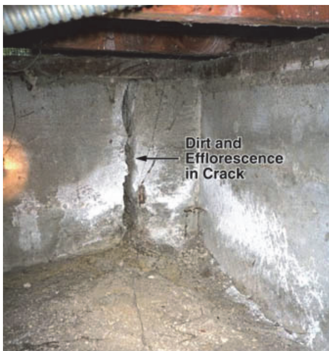
Figure 6-14 Dirt and efflorescence indicates age of foundation wall crack is not recent (photo credit: Exponent).
