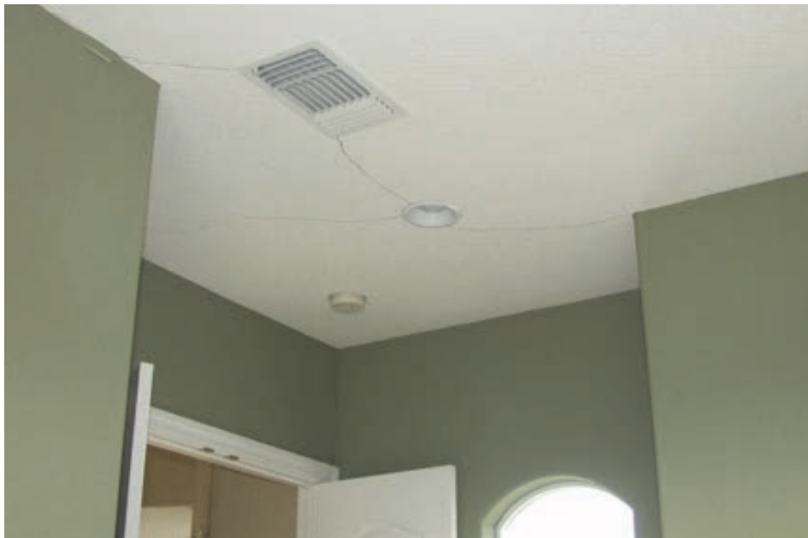
Figure 2-37 Cracking of ceiling finishes caused by the 2003 San Simeon, California earthquake (photo credit: Exponent).
