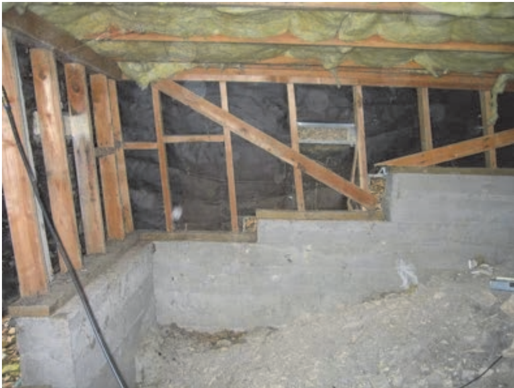
Figure 2-5 Damaged framing enclosing the underfloor area of a hillside house caused by the 2003 San Simeon, California earthquake. The damage includes detachment of the stucco from the wall framing and both in-plane racking and out-of-plane leaning of the wood-frame walls (photo credit: Exponent).
