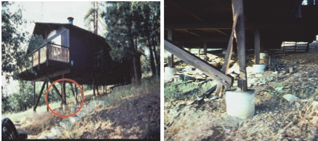
Figure 2-35 Damage at bolted connection of diagonal lumber bracing to post at hillside house. Damage at the connection includes splitting of the diagonal lumber brace and fracture of the post (photo credit: R. Gallagher).
