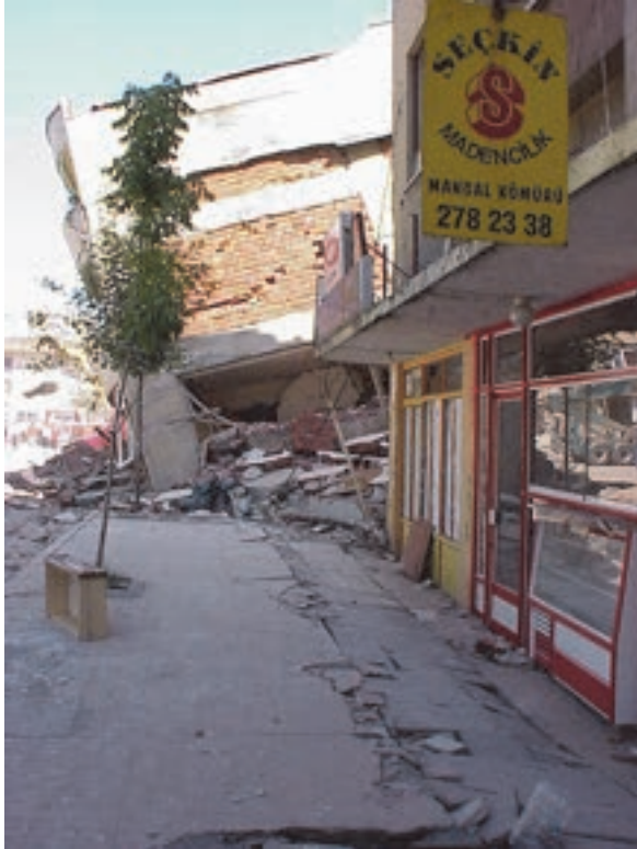
Figure 5-14 Settlement relative to surrounding ground (foreground) of mat foundation in Adapazari from the 1999 Kocaeli, Turkey earthquake (photo credit: J. P. Stewart).
