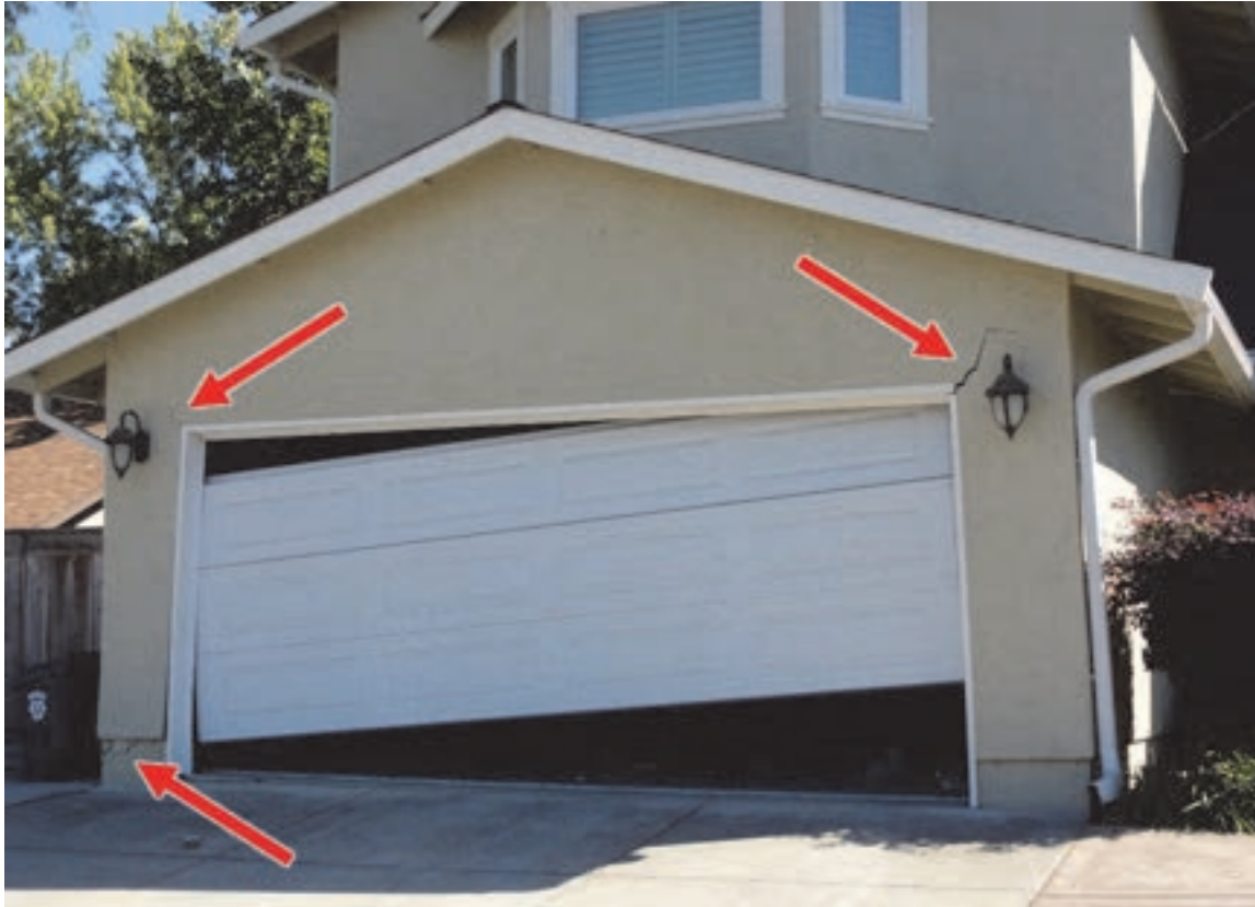
Figure 2-8 Damage related to living space over garage caused by the 2014 South Napa, California earthquake. In-plane racking of the front wall line of the garage caused cracking and possible framing damage in the narrow wall segments on either side of the garage door (photo credit: Exponent).
