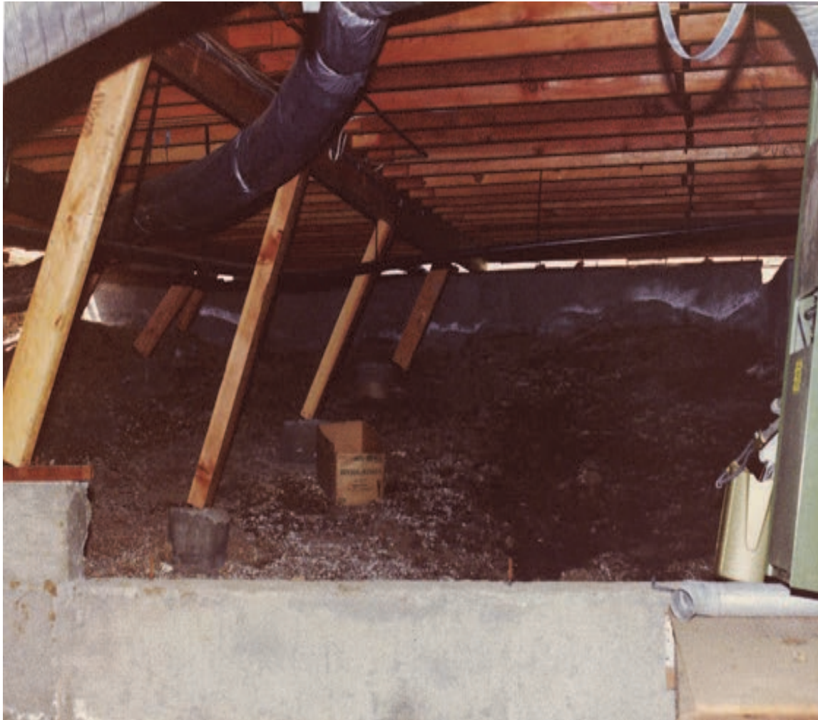
Figure 2-14 Leaning posts within the interior of the house plan. The house had a perimeter foundation with inadequate anchorage between the superstructure and the foundation (photo credit: R. Gallagher).
