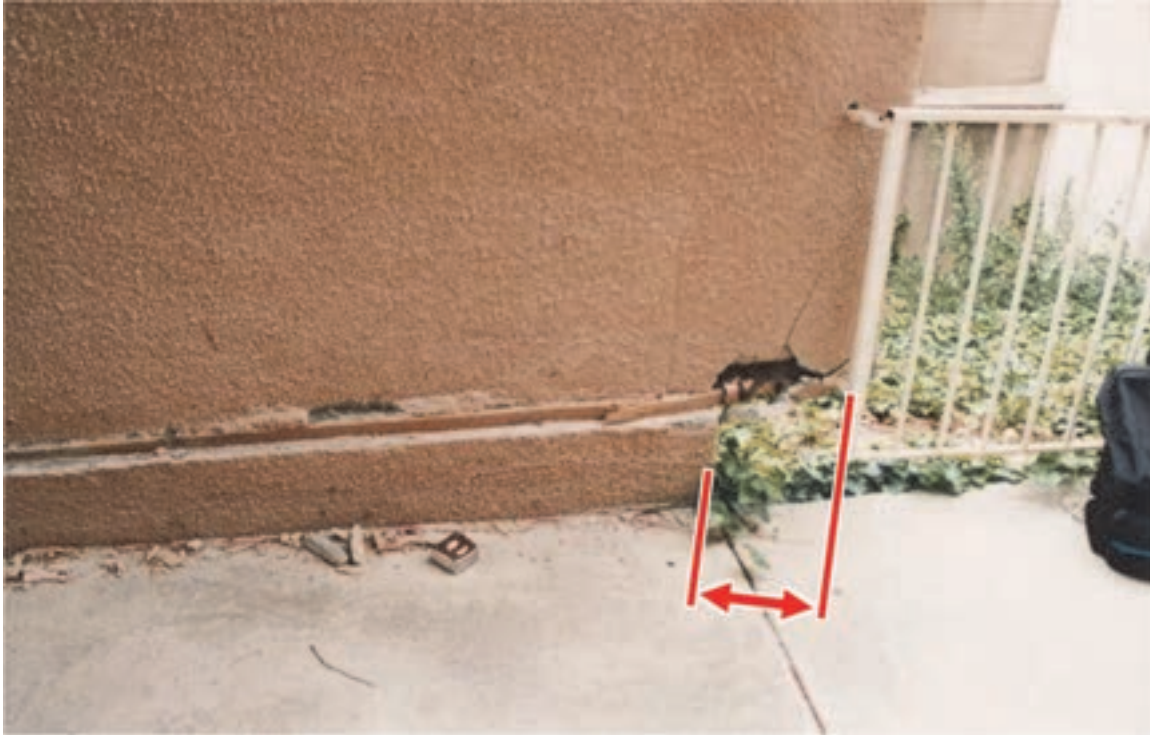
Figure 2-1 Earthquake-caused sliding of superstructure at foundation. The wall has shifted to the right several inches relative to the foundation, stucco wall finishes have cracked and spalled along the sill plate, and the sill plate is fractured near the right end of the wall (photo credit: Exponent).
