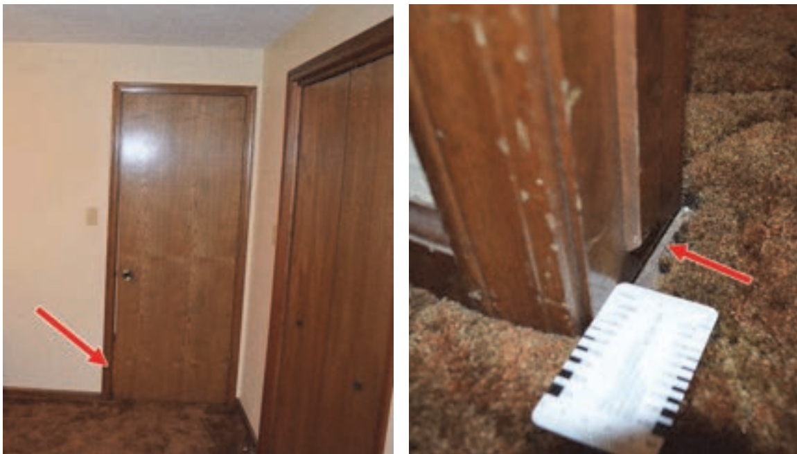
Figure 2-2 Earthquake-caused sliding of superstructure at floor slab. The wall has shifted less than 1 inch to the left, as evidenced in the left photo by the tapered gap between the left side of the door and doorjamb and in the right photo by the gap between the carpet and doorjamb (photo credit: Exponent).
