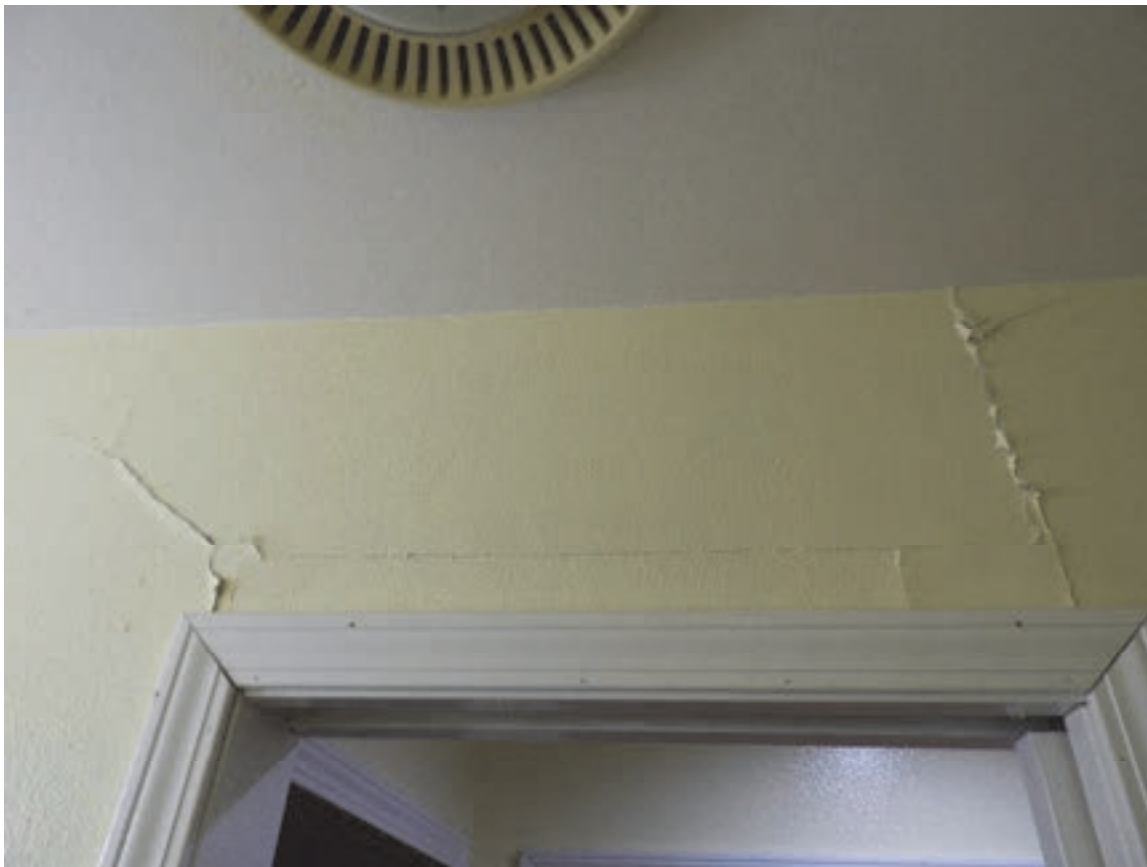
Figure 2-27 Cracking of gypsum wallboard at corners of door opening caused by the 2018 Anchorage, Alaska earthquake (photo credit: Z. Stutts).
