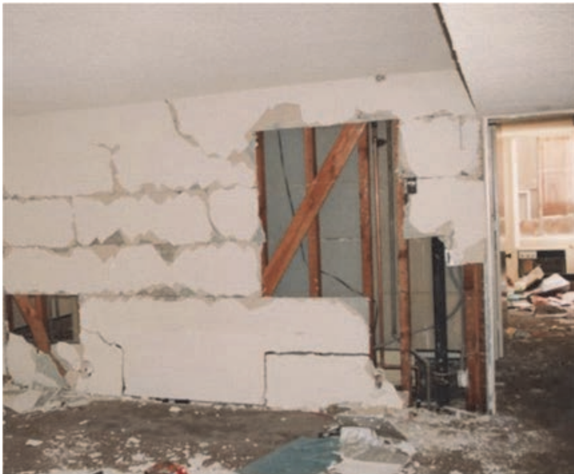
Figure 2-26 Earthquake-induced cracking and delamination of plaster on gypsum lath (photo credit: Exponent).
