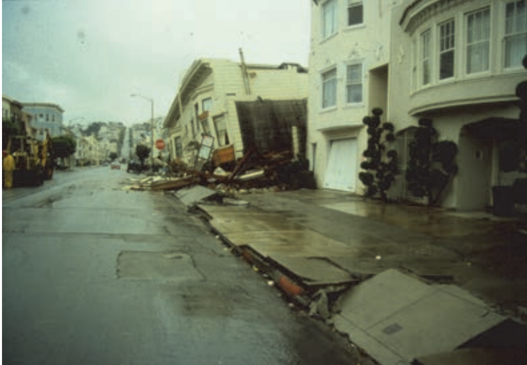
Figure 5-7 Buckled pavement from liquefaction-induced ground oscillations, San Francisco Marina District, 1989 Loma Prieta, California earthquake (Seed et al., 1990).
