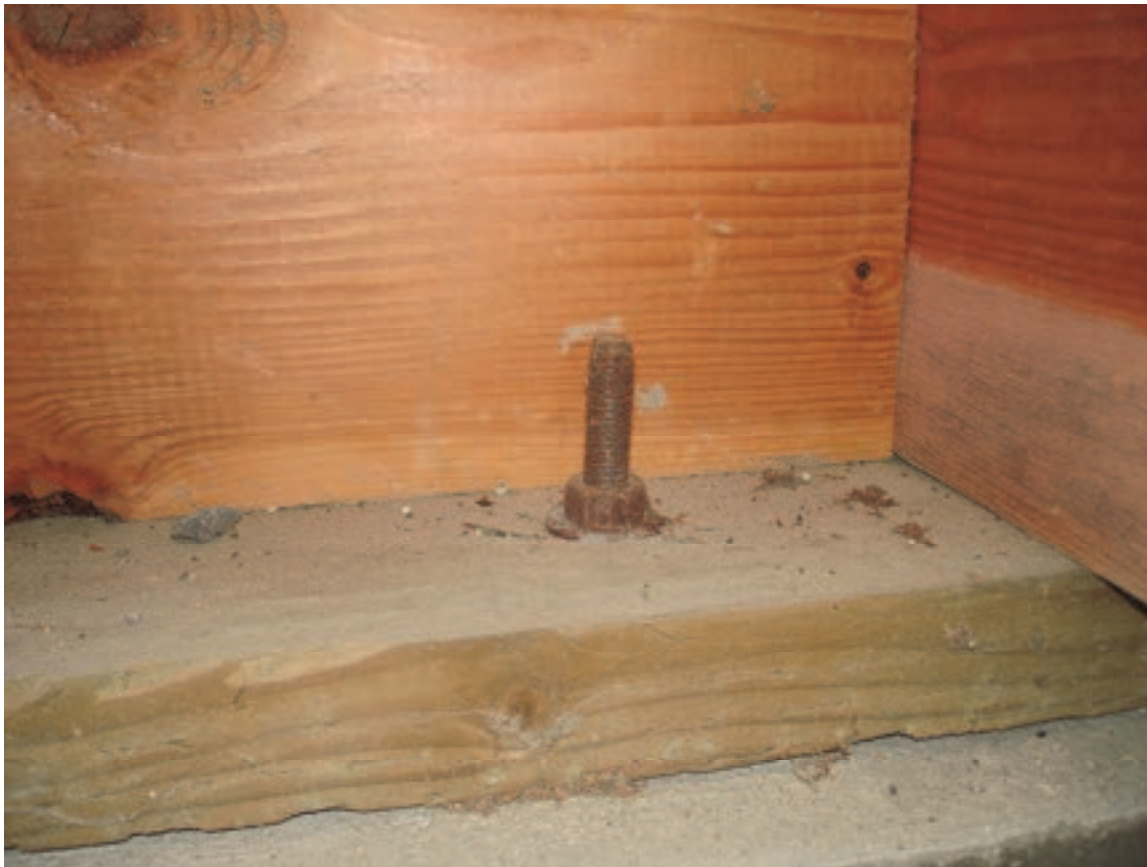
Figure 2-18 Typical steel cast-in-place anchor bolt attaching sill plate to concrete foundation (photo credit: E. Mikailian).
