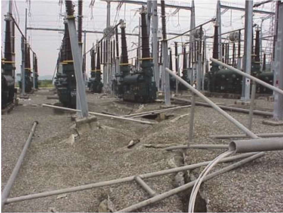
Figure 5-20 Head scarp of coherent landslide at Junliau Switching Station, Taiwan, induced by 1999 Chi Chi, Taiwan earthquake. Slide movements of approximately 3 feet to 4 feet occurred along a bedding plane in rock (photo credit: J. P. Stewart).
