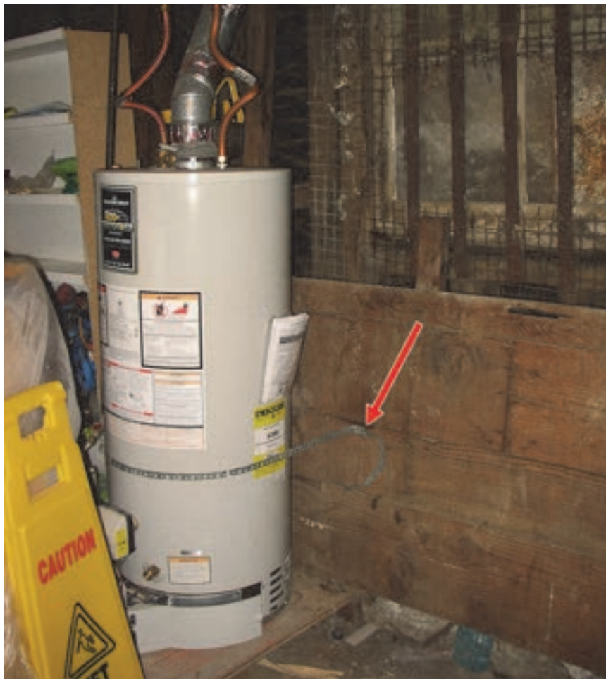
Figure 2-40 Inadequately strapped water heater (photo credit: D. Bonowitz).
