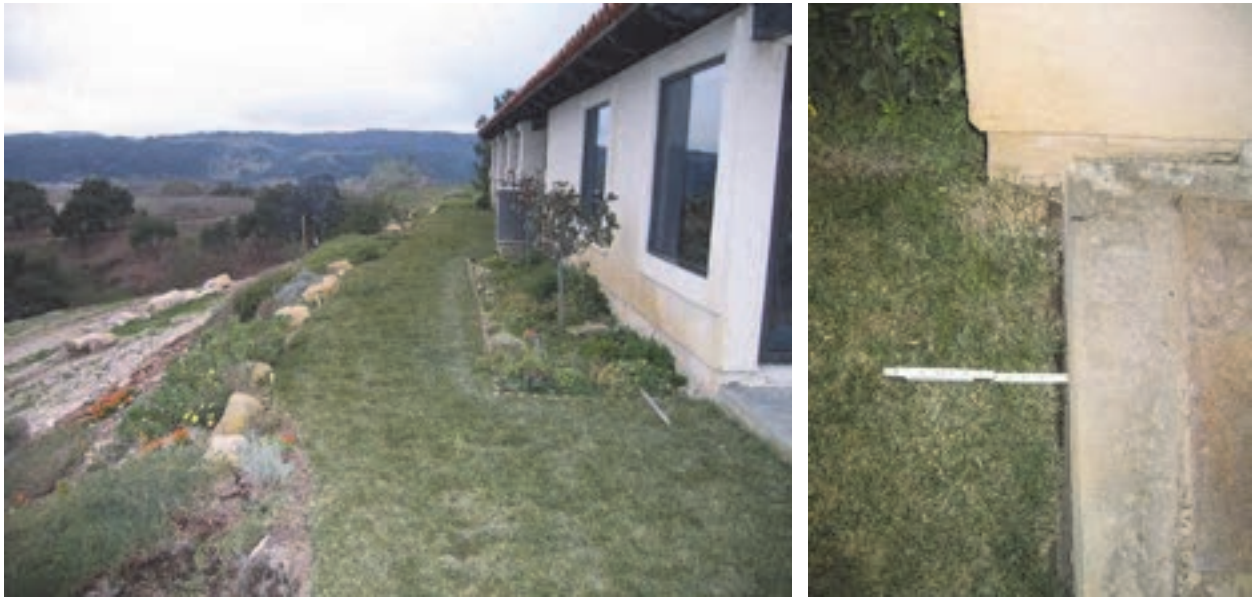
Figure 6-15 Ground separation from residence along slope side of structure following the 2003 San Simeon, California earthquake (image credit: Exponent).
