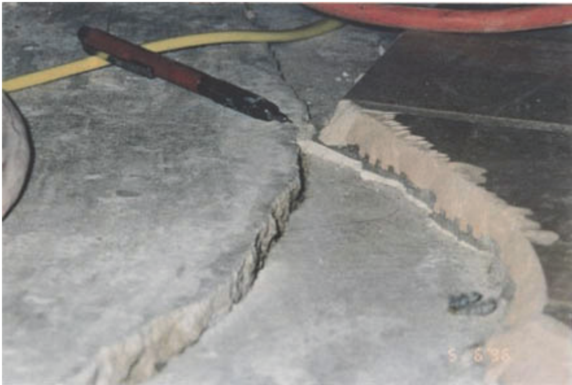
Figure 6-12 Grout completely filling the slab-on-grade crack (indicated by pencil) indicates that slab crack was present at the time of the tile installation and has not experienced movement since tile installation (photo credit: Exponent).
