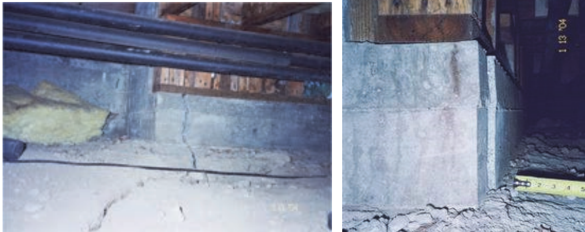
Figure 2-11 Cracking of concrete stemwall in-line with ground crack resulting from the 2003 San Simeon, California earthquake (left). The offset across the crack is revealed in the photograph on the right (photo credit: Exponent).
