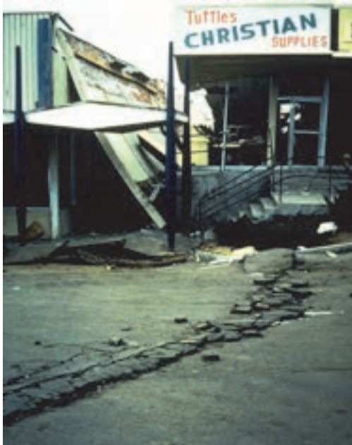
Figure 5-1 Surface fault rupture from the 1971 San Fernando, California earthquake and associated damage to pavement and structures in the Sylmar area (photo credit: National Information Service for Earthquake Engineering, or NISEE).
