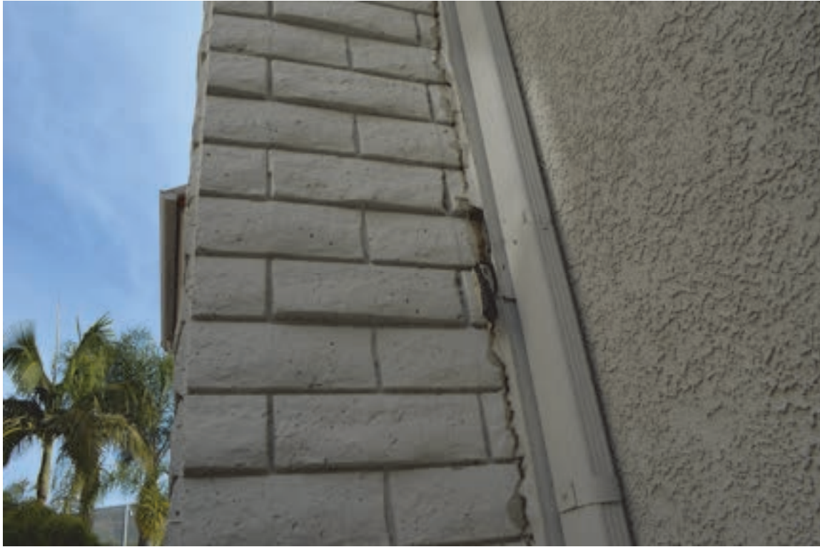
Figure 2-39 Separation of chimney from house caused by the 2014 La Habra, California earthquake. The separation was relatively minor, and the chimney remained attached to the house (photo credit: Exponent).
