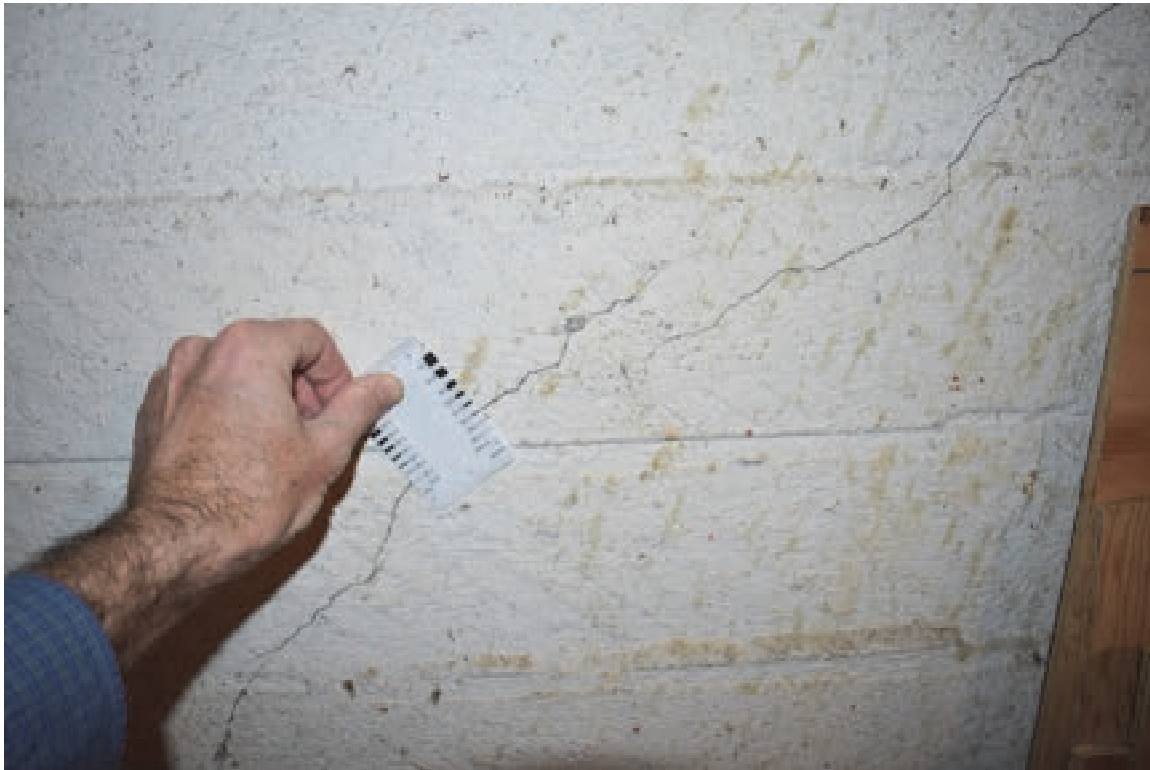
Figure 2-15 Typical non-earthquake-related cracking of concrete California basement wall (photo credit: Exponent).
