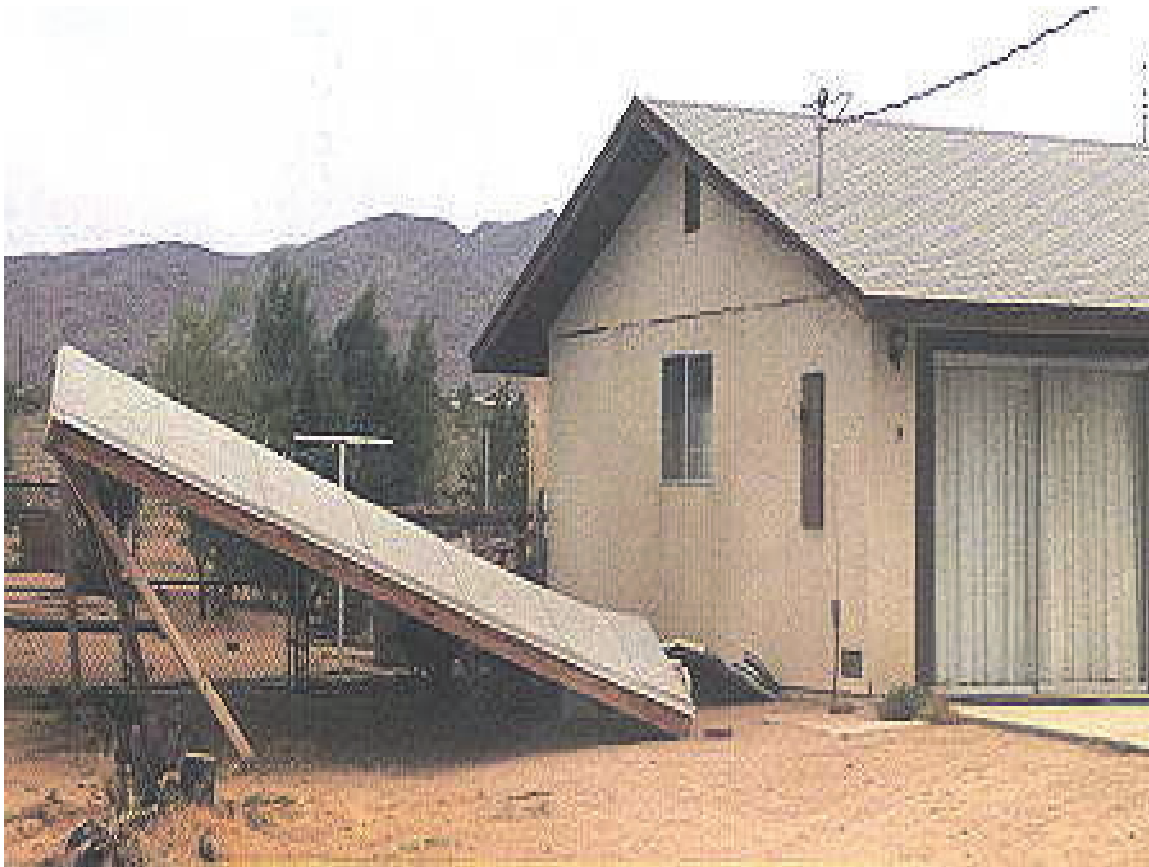
Figure 2-42 Earthquake-caused detachment of the carport from the house wall, resulting in collapse (photo credit: California Office of Emergency Services).
