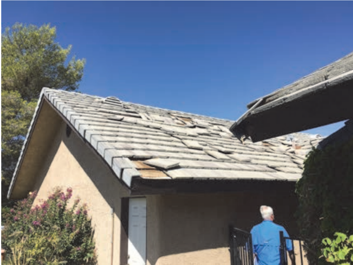
Figure 2-41 Displaced roof tiles caused by the 2019 Ridgecrest, California earthquake (photo credit: M. Ziemer).
