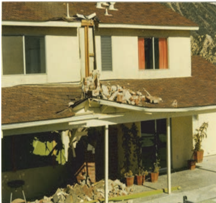
Figure 2-36 Damage to porch roof framing caused by chimney collapse (photo credit: R. Gallagher).
