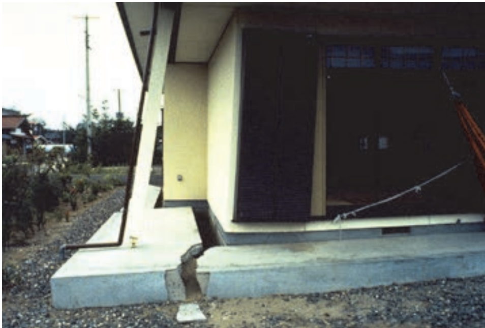
Figure 6-4 Damage to house foundation in Wakami, Japan, caused by lateral spreading following the 1983 Nihonkai-Chubu, Japan earthquake (photo credit: NISEE).
