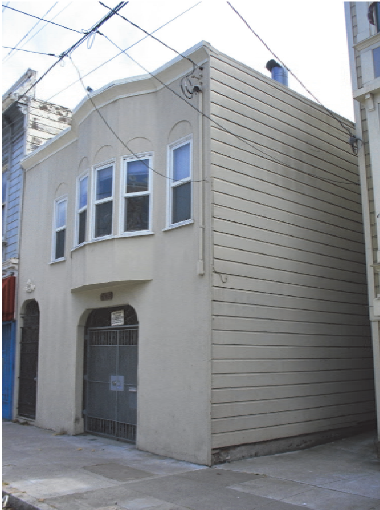
Figure 2-22 Horizontal wood siding (shiplap) on the side wall and stucco on the front face of a house with a living-space-over-garage condition (photo credit: D. Bonowitz).
