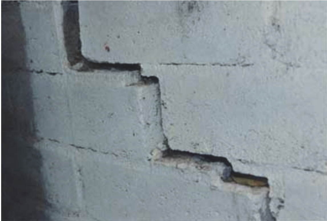
Figure 6-13 Paint within concrete block wall crack indicates that the crack was present at the time of last painting (photo credit: Exponent).
