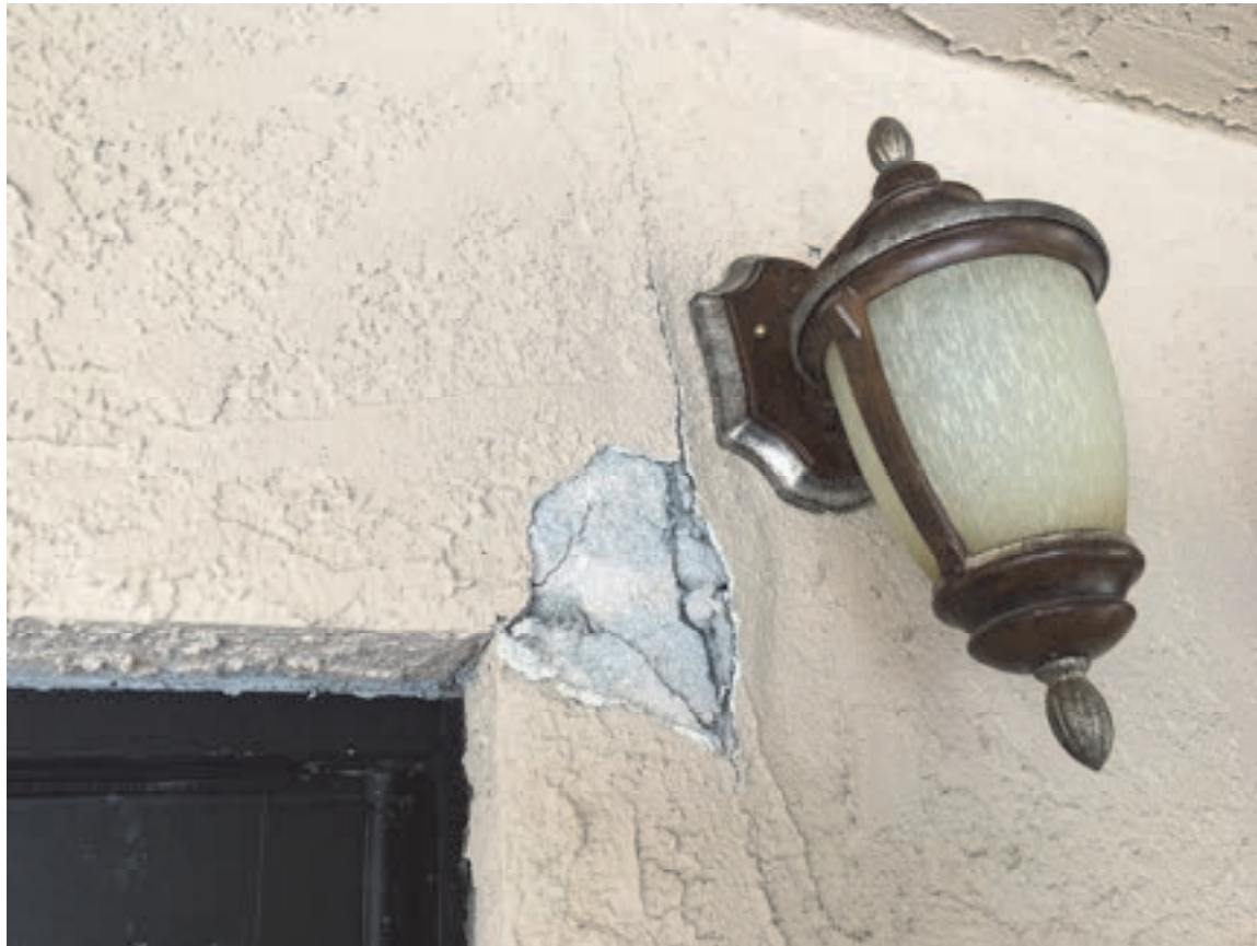
Figure 2-24 Stucco cracking and spalling at a door opening due to the 2019 Ridgecrest, California earthquake (photo credit: M. Ziemer).
