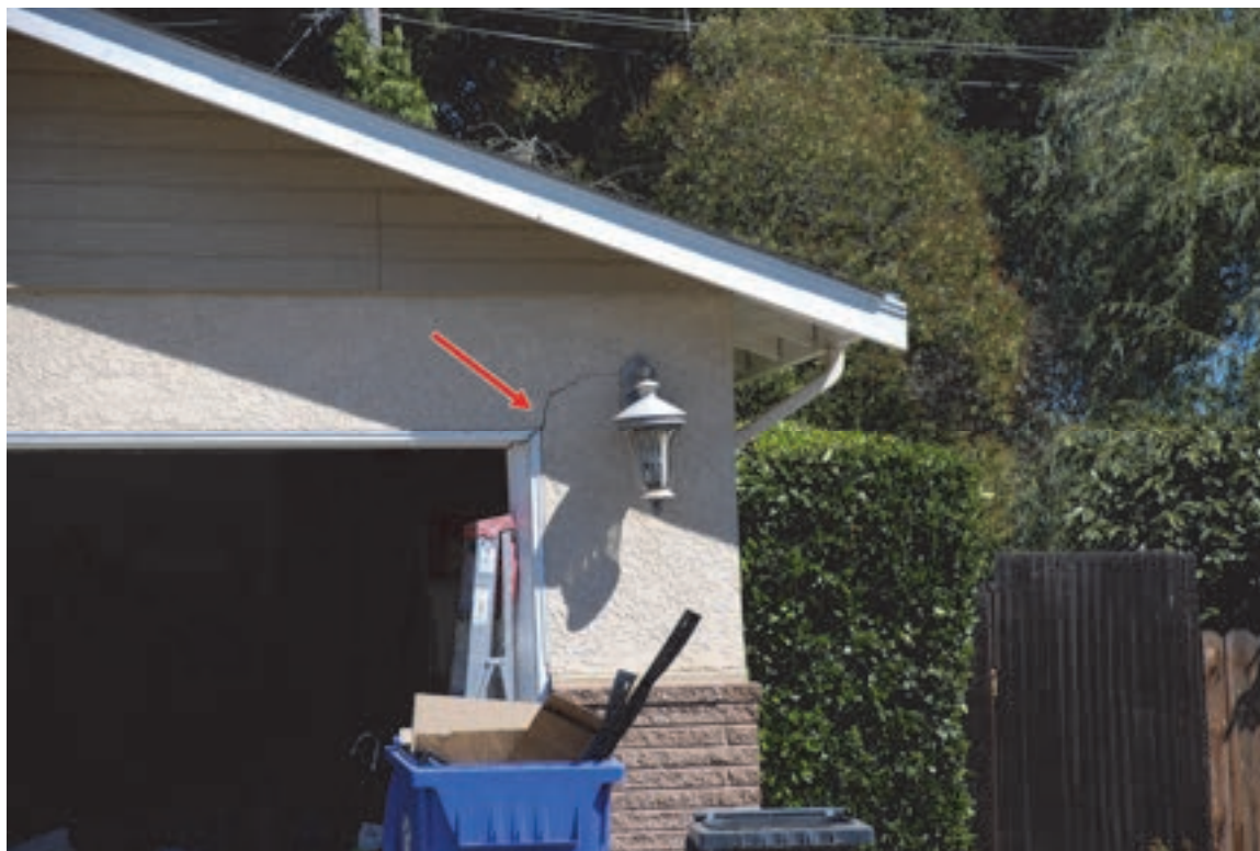
Figure 2-33 Concentrated earthquake damage to stucco at the top of a narrow wall segment adjacent to a garage door (photo credit: K. Cobeen).
