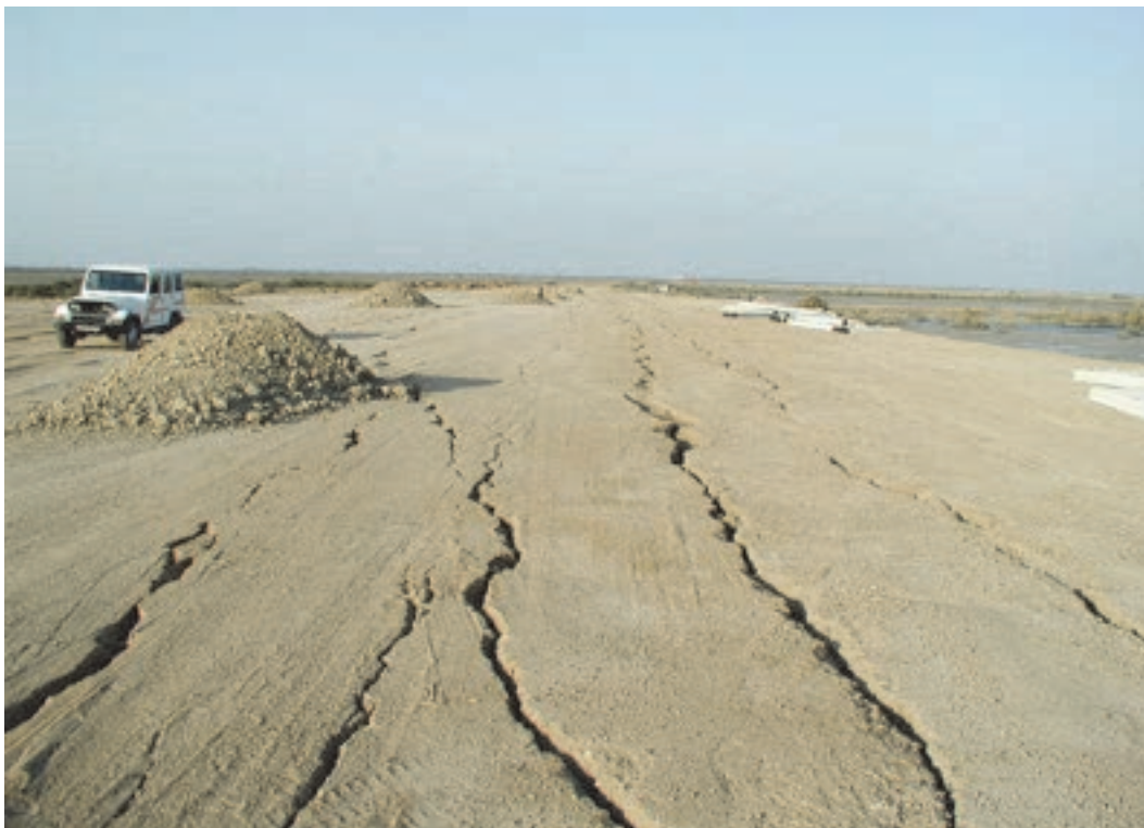
Figure 5-8 Ground cracking of fill from liquefaction-induced cyclic mobility of foundation soils during 2001 Gujarat, India earthquake (photo credit: J. P. Stewart).
