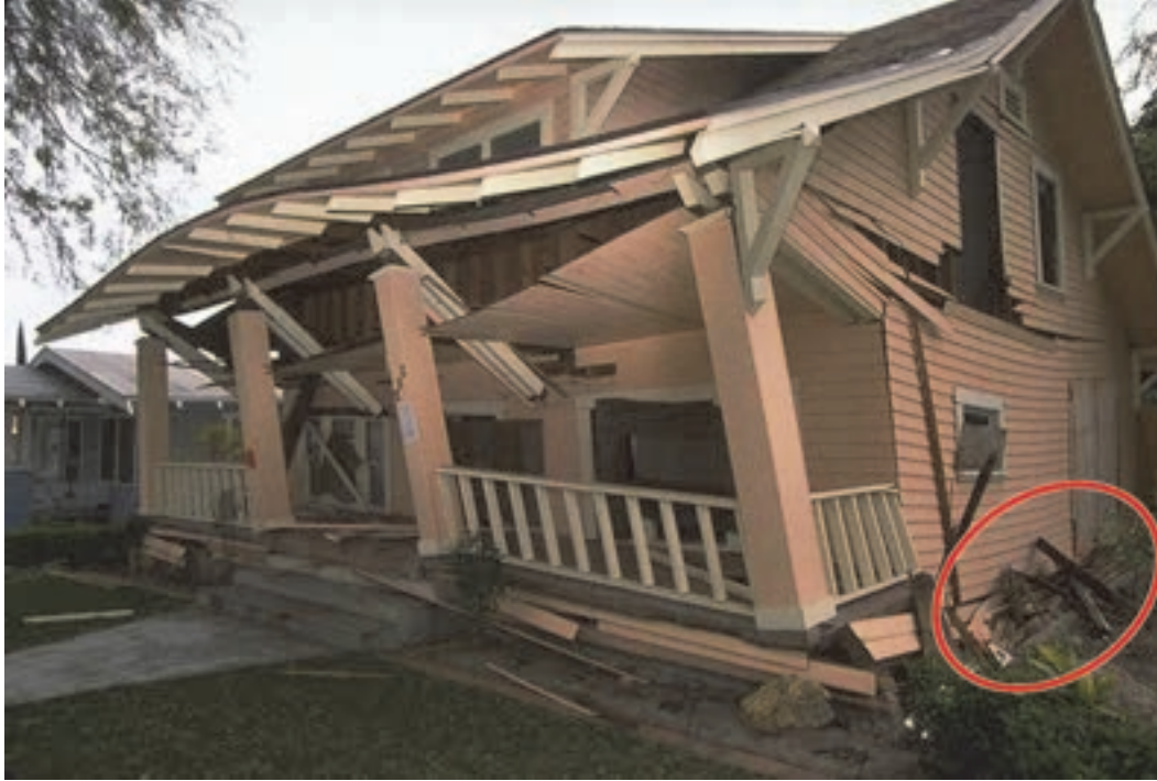
Figure 2-4 Cripple wall collapse caused by the 1994 Northridge, California earthquake resulting in widespread related damage in upper-story framing and relative movement between the main house and the covered porch (photo credit: Federal Emergency Management Agency, or FEMA).
