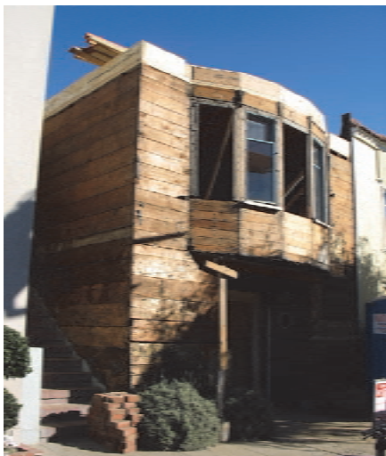
Figure 2-30 Horizontal lumber sheathing revealed by the removal of exterior finishes (photo credit: D. Bonowitz).
