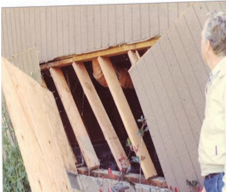
Figure 2-23 Plywood panel siding detached from cripple wall framing at a hillside house (photo credit: R. Gallagher).
