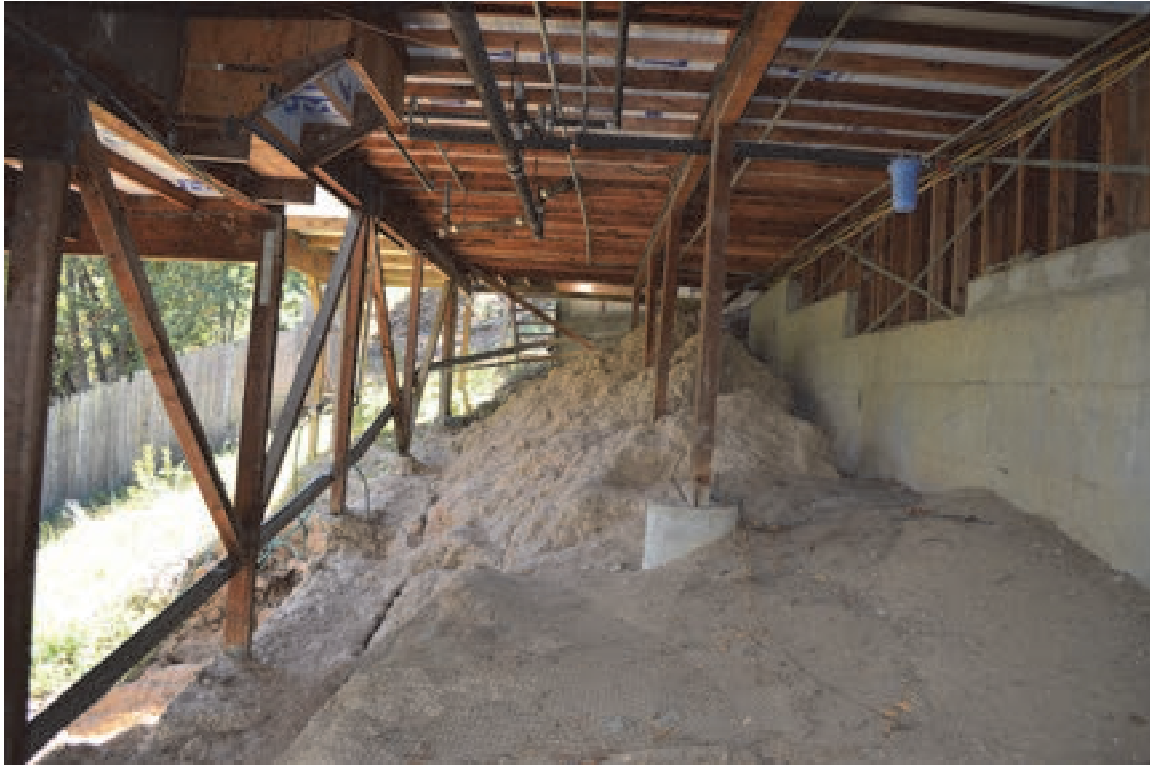
Figure 2-21 View of the framing connections to the uphill foundation (at right side of the photograph) at a hillside house (photo credit: Exponent).
