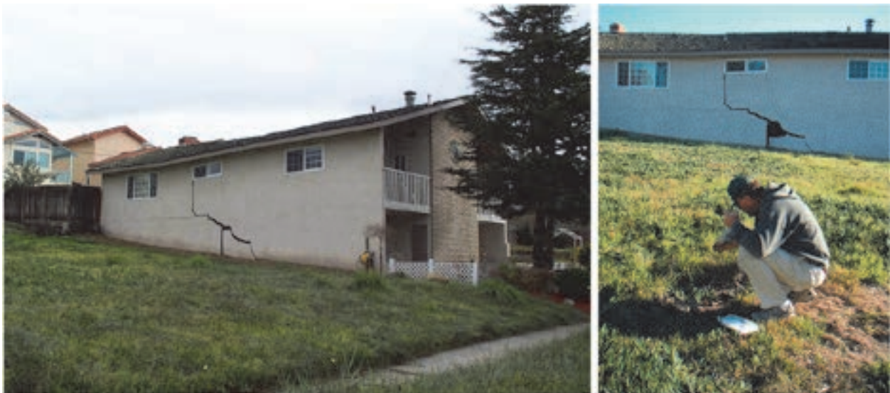
Figure 5-15 Damage to a residence in Oceano, California from lateral spreading following the 2003 San Simeon earthquake. Photo (right) taken along head scarp offset and its intersection with residence foundation (photo credits: San Luis Obispo County Department of Planning & Building, left; Holzer et al., 2004, right).
