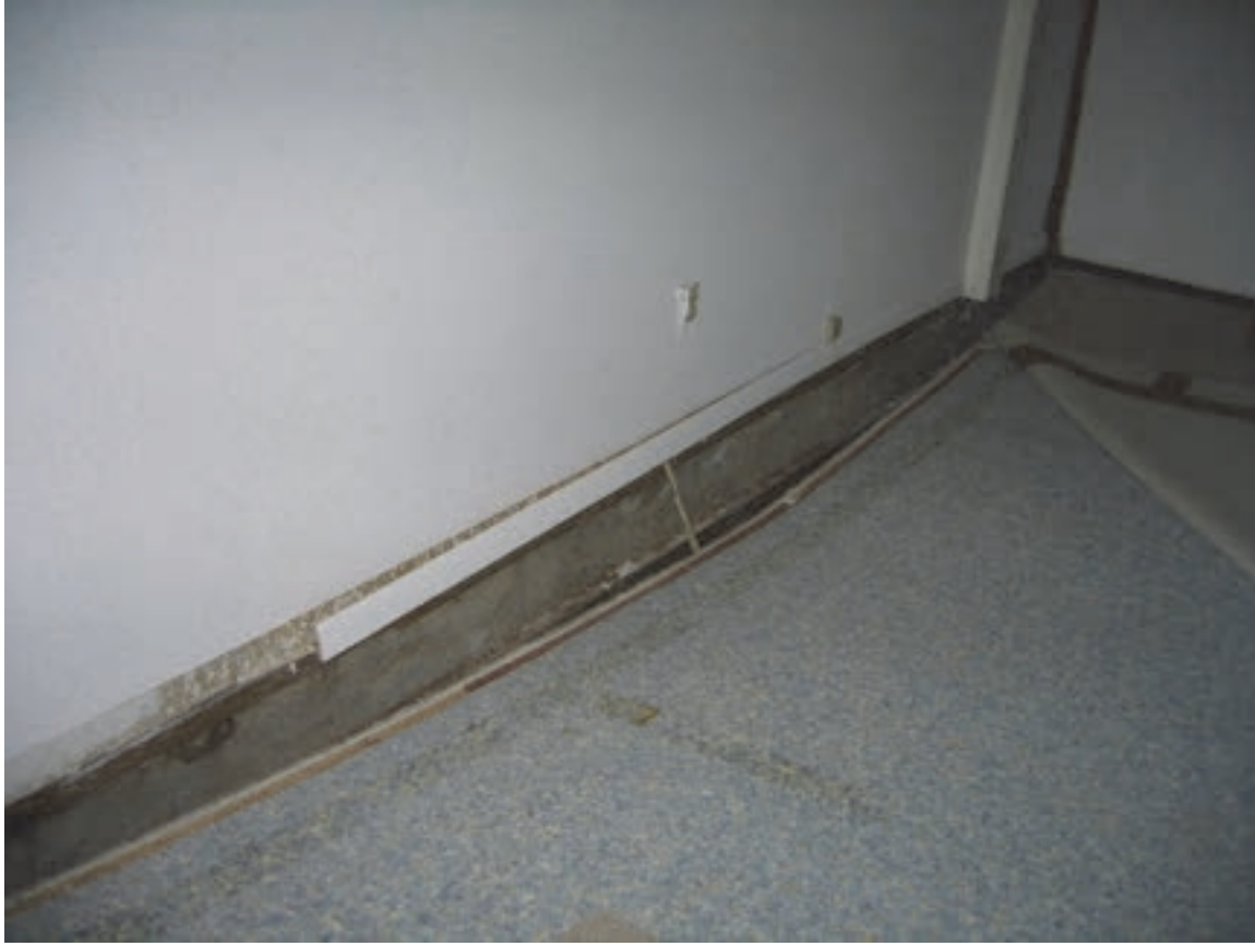
Figure 2-6 Damage at uphill end of a hillside house caused by the 2003 San Simeon, California earthquake. The floor framing detached and pulled away from the uphill foundation, causing the floor to sag (photo credit: Exponent).
