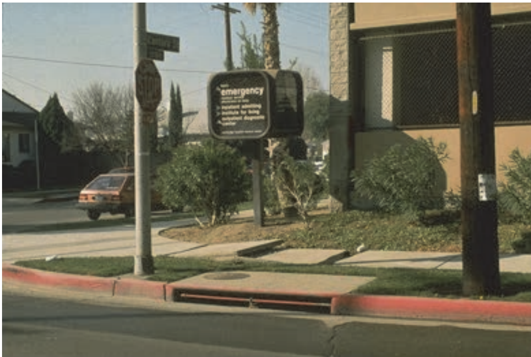
Figure 6-7 Sidewalk buckled from lateral compression by the Northridge Hospital Medical Center from the 1994 Northridge, California earthquake (photo credit: NISEE).
