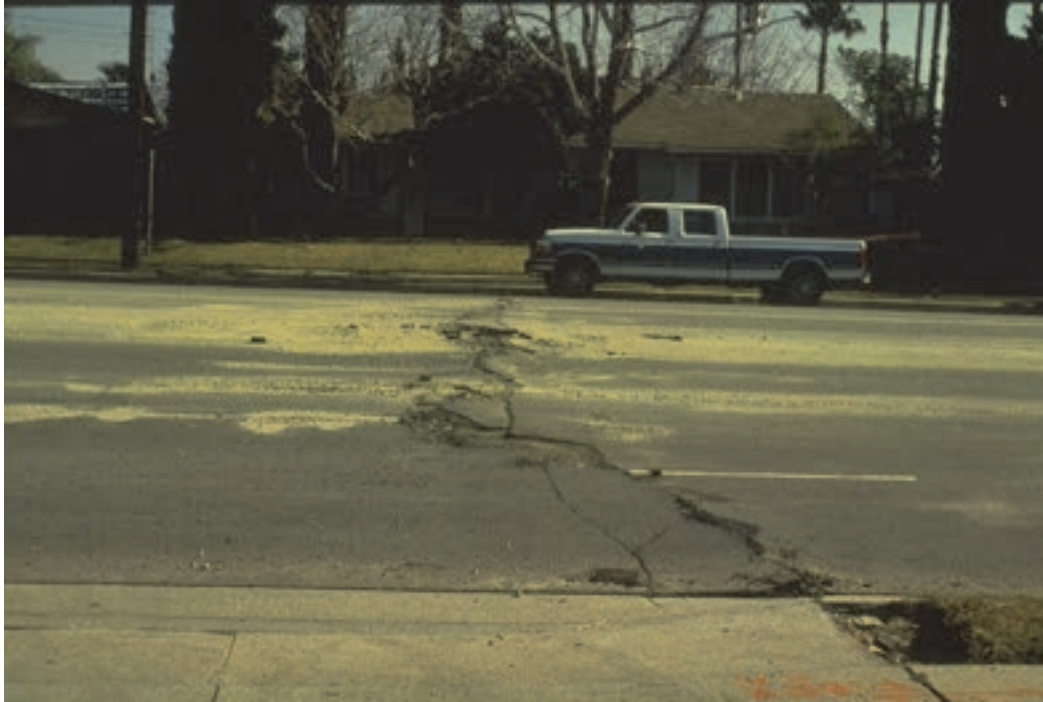
Figure 6-6 Localized compression feature and pavement damage from the 1994 Northridge, California earthquake (photo credit: NISEE).
