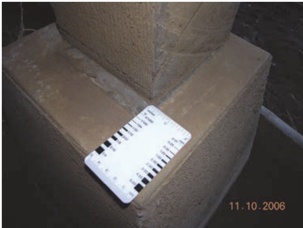
Figure 2-13 Shifting of an unattached wood post along the top of the concrete pier due to the 2006 Kiholo Bay, Hawaii earthquake. There was no continuous perimeter foundation around the building (photo credit: Exponent).
