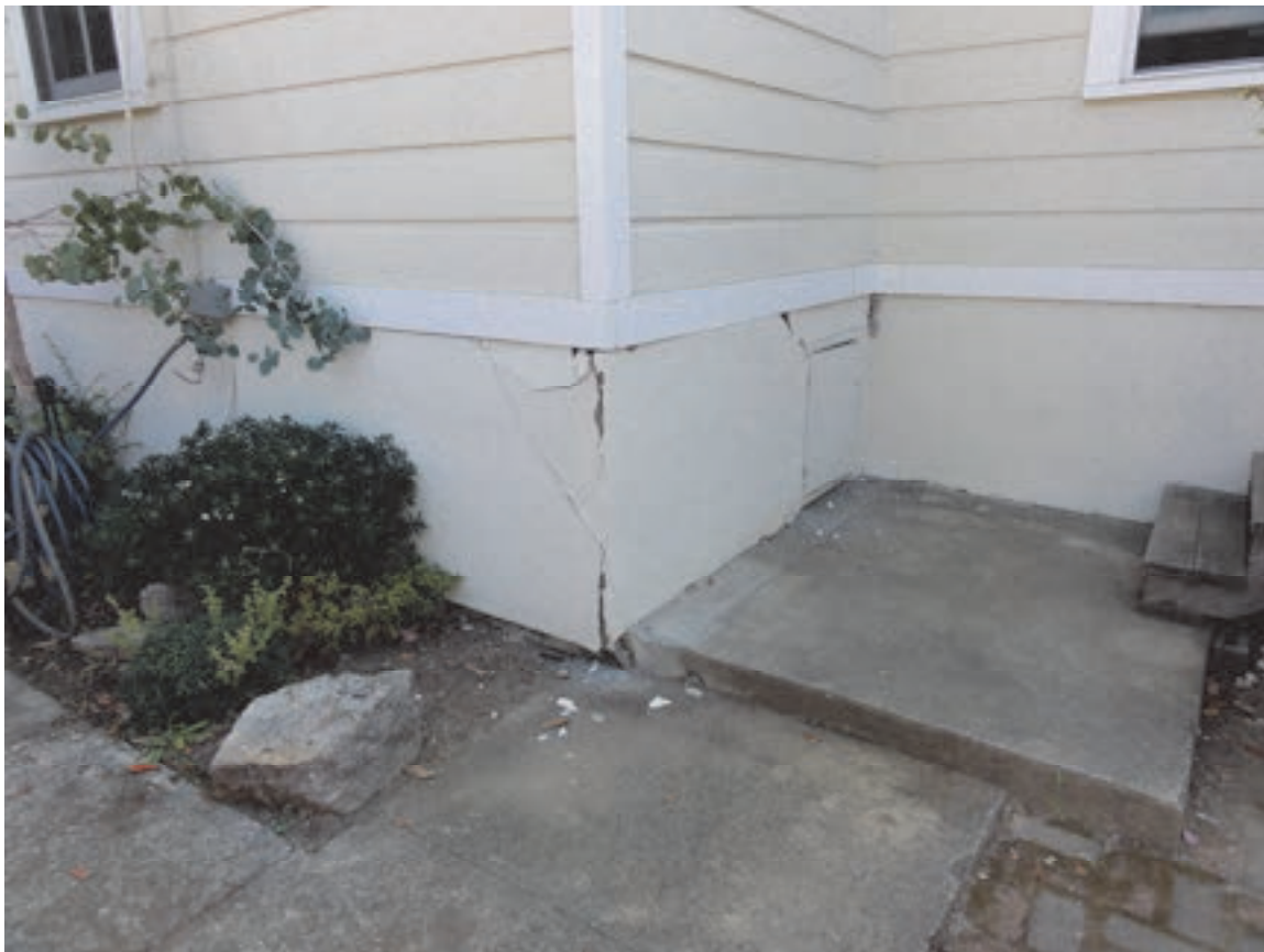
Figure 2-3 Damage to cripple wall finishes caused by the 2014 South Napa, California earthquake (photo credit: Exponent).
