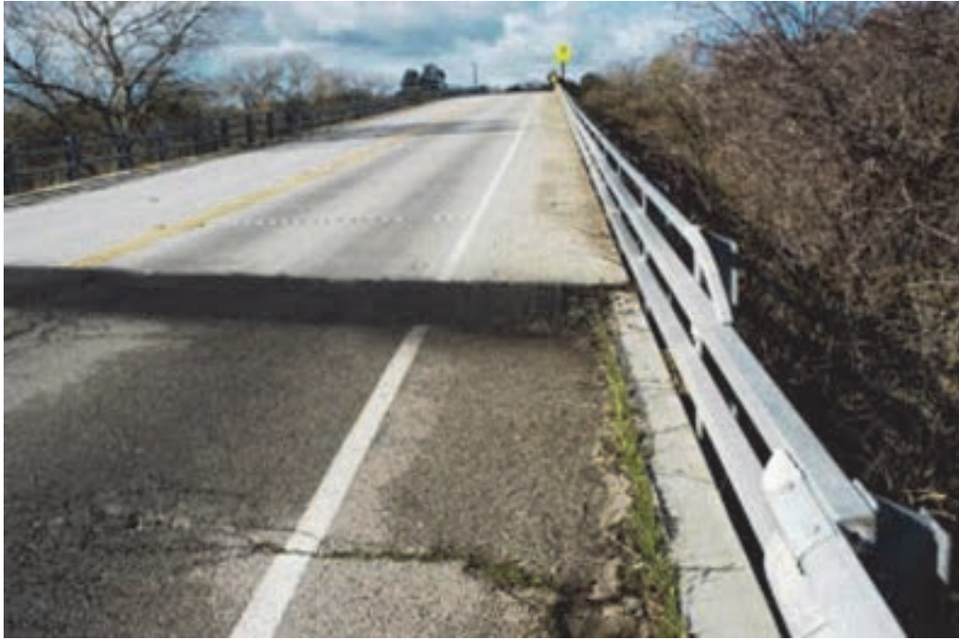
Figure 5-11 Templeton Road Bridge settlement following the 2003 San Simeon, California earthquake. The settlement of approximately 5 inches was a result of liquefaction beneath the bridge abutment foundation (EERI, 2004).
