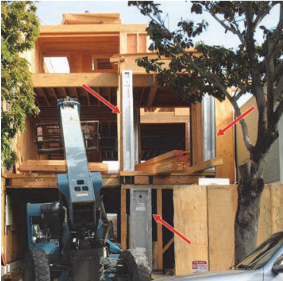
Figure 2-34 Proprietary shear walls at narrow wall piers between large window and door openings (photo credit: D. Bonowitz).
