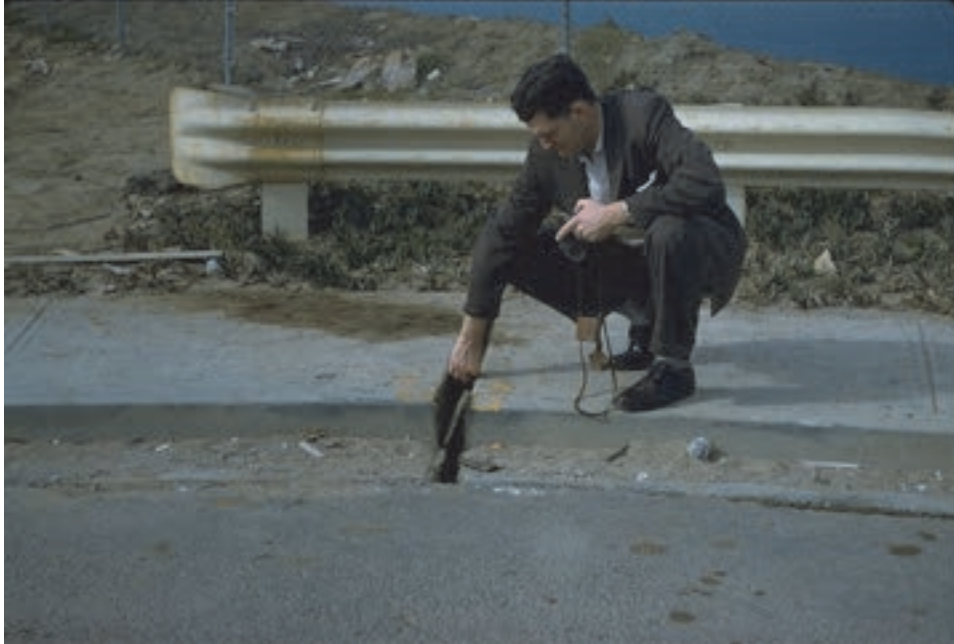
Figure 6-3 Separation in sidewalk from 1957 Daly City, California earthquake (photo credit: NISEE).
