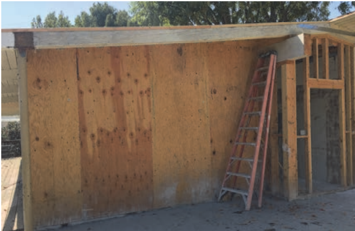
Figure 2-28 Wood structural panel (plywood) sheathing revealed by the removal of exterior finishes (photo credit: E. Mikailian).
