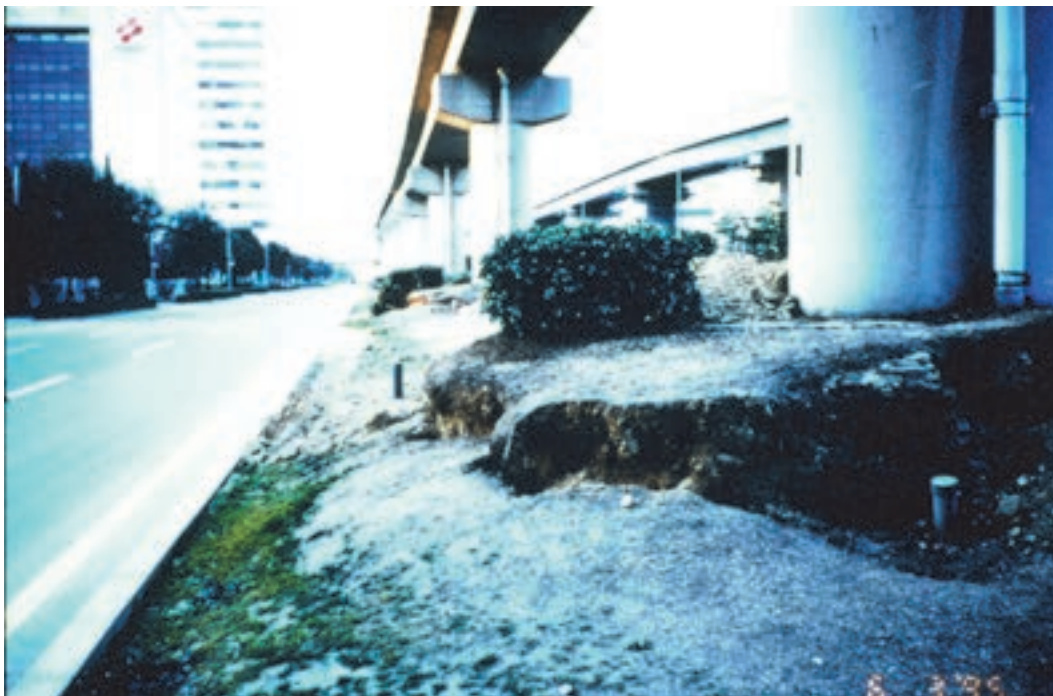
Figure 5-10 Uniform settlement of liquefied fill soils, 1995 Kobe, Japan earthquake. The amount of settlement is shown by the difference between the unsettled pile-supported bridge bent and the surrounding ground. The uniformity of the settlement is shown by the lack of cracking in the pavement (Sitar et al., 1995).
