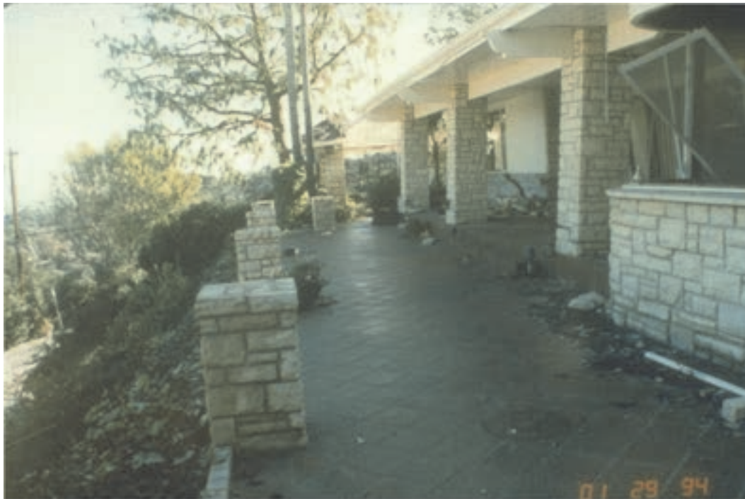
Figure 5-16 Structure damaged by movements in wedge fill from the 1994 Northridge, California earthquake (photo credit: NISEE).
