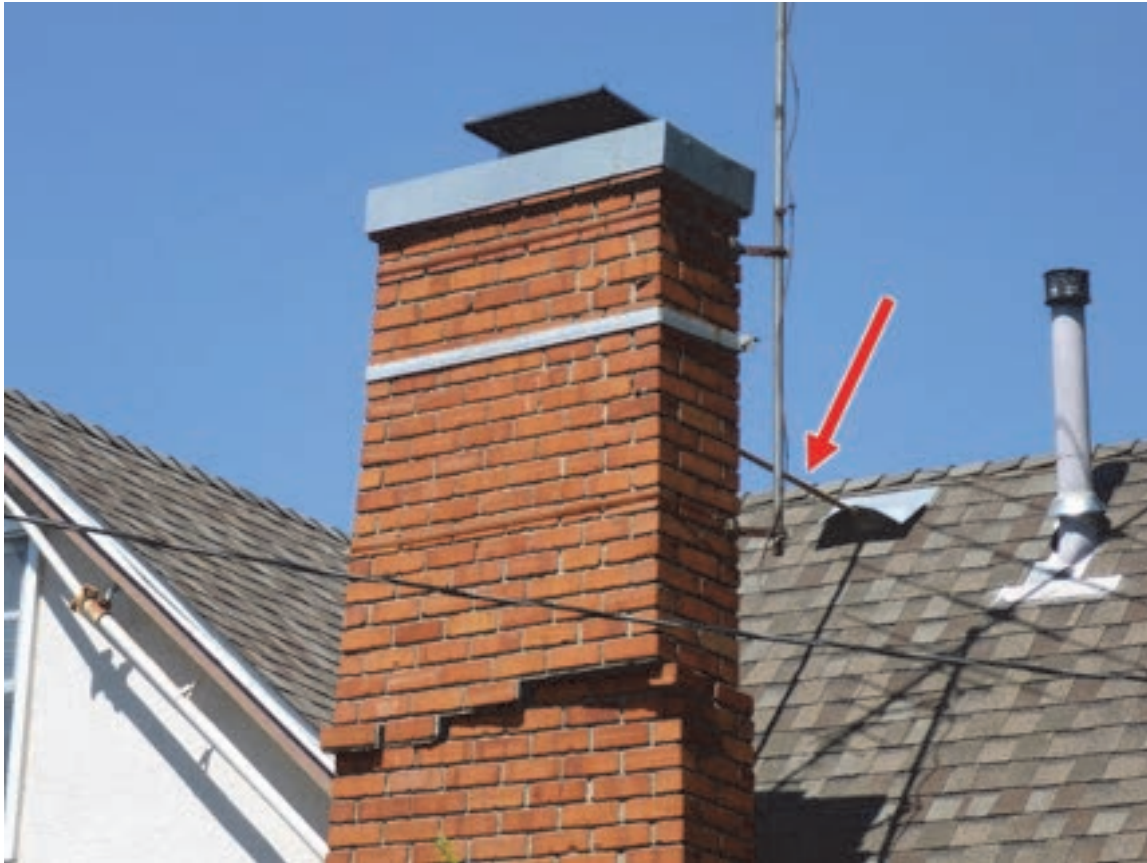
Figure 2-38 Earthquake-induced fractured chimney near the roof line. The brace between the chimney and roof, visible behind the chimney, was not adequate to prevent the damage (photo credit: Exponent).
