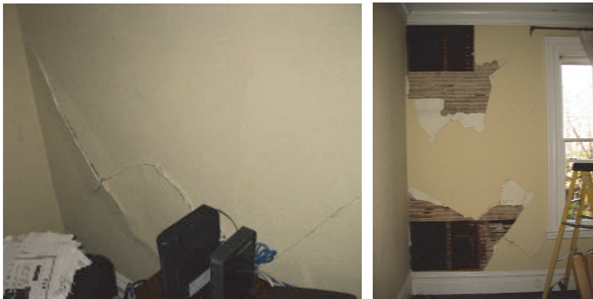
Figure 2-25 Detachment of plaster from wood lath (left) with destructive investigation (right) revealing that the wood framing had not sustained earthquake damage (photo credit: D. Bonowitz).
