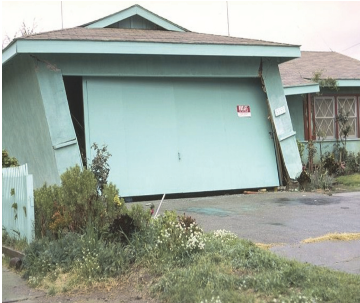
Figure 2-7 Large in-plane drift of narrow wall piers at garage door opening caused by the 1971 San Fernando, California earthquake (photo credit: National Information Service for Earthquake Engineering, or NISEE).
