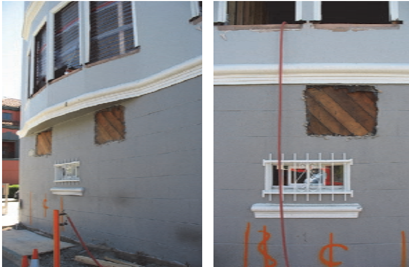
Figure 2-29 Diagonal lumber sheathing revealed by the removal of exterior finishes (photo credit: D. Bonowitz).
