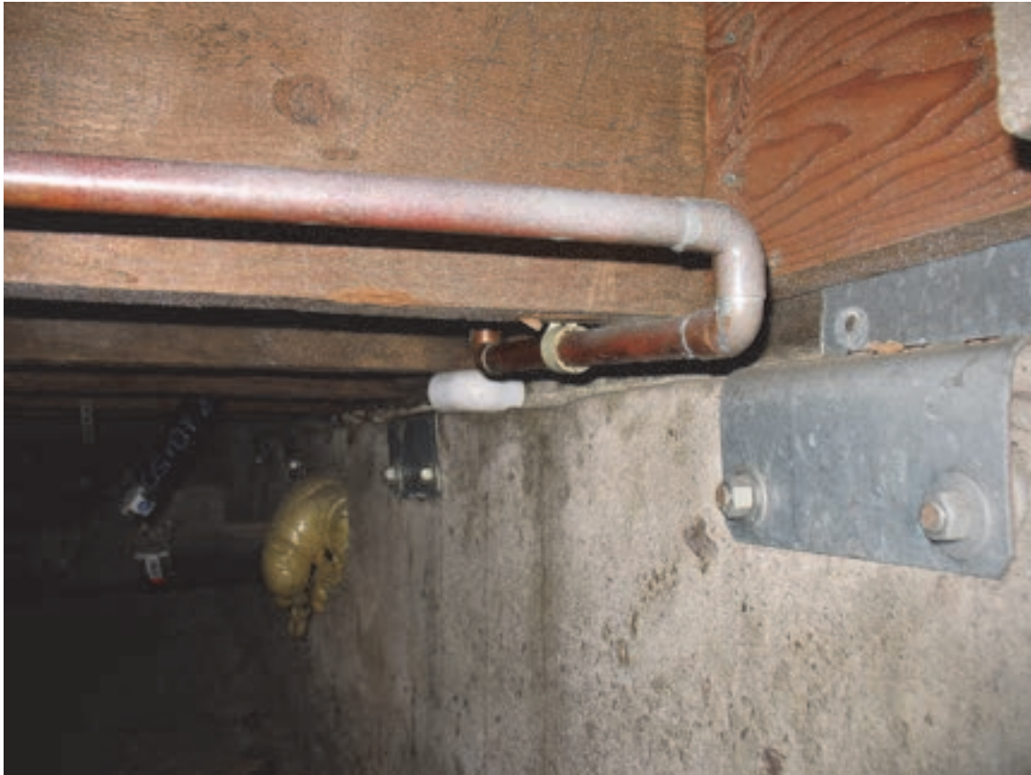
Figure 2-20 Steel post-installed plate connectors attaching a wood sill plate to a concrete stemwall. The connectors were installed as part of a seismic retrofit (photo credit: D. Bonowitz).
