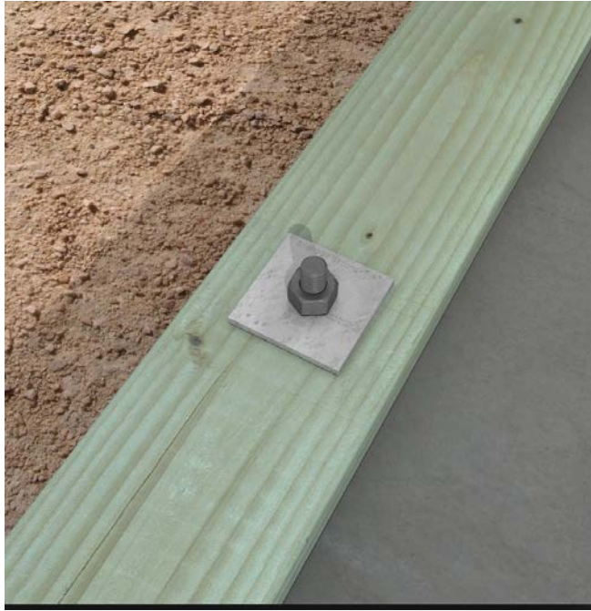
Photo: A square washer absorbs movement (converting it into an upward pull on the plate) and acts to prevent splitting of the mudsill.
