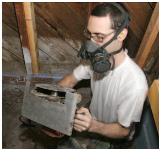
Figure 12. Using a saw equipped with a flush-cutting attachment (left), a carpenter trims the mudsill back to the stud plane (below). This makes for a stronger shear wall because the bottom edge of plywood nails directly to the mudsill. The alternative is to nail the plywood to short blocks installed between the studs.
