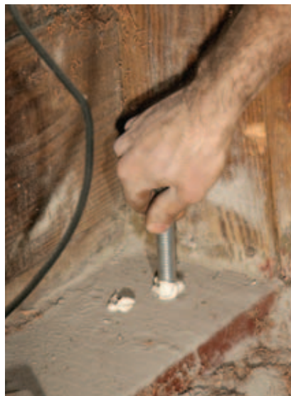
Figure 10. After drilling a hole for a hold-down, a carpenter blows it clean with compressed air (top left). He knocks loose material from the sides by reaming it with a long wire brush (top right), then blows it out again. He finishes by pumping two-part epoxy into the hole (above left) and inserting a length of threaded rod (above right). Once the epoxy sets, he will bolt in the hold-down and sheathe the wall with plywood.
