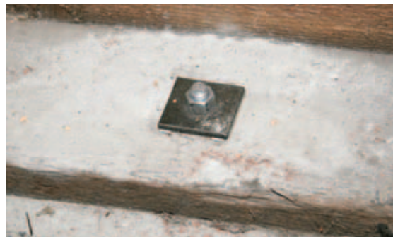
Figure 6. The author's crew typically adds anchor bolts to prevent mudsills from sliding horizontally in an earthquake. Bolts perform better when they are installed with 2-inch-by-2-inch washer plates.
