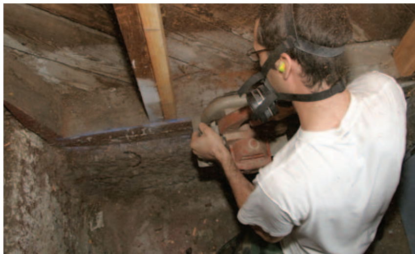
Figure 12. Using a saw equipped with a flush-cutting attachment (left), a carpenter trims the mudsill back to the stud plane (below). This makes for a stronger shear wall because the bottom edge of plywood nails directly to the mudsill. The alternative is to nail the plywood to short blocks installed between the studs.
