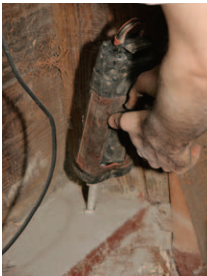
Figure 10. After drilling a hole for a hold-down, a carpenter blows it clean with compressed air (top left). He knocks loose material from the sides by reaming it with a long wire brush (top right), then blows it out again. He finishes by pumping two-part epoxy into the hole (above left) and inserting a length of threaded rod (above right). Once the epoxy sets, he will bolt in the hold-down and sheathe the wall with plywood.
