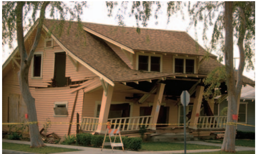
Figure 2. The building at top slid off its foundation during a magnitude-6.5 earthquake in 2004. The house itself is in pretty good shape and would have likely survived unscathed if the cripple walls and foundation attachments had been reinforced. The cripple walls under the house above collapsed during the Northridge earthquake, causing serious structural damage. With damage this severe, it's usually cheaper to tear the house down than to repair it.
