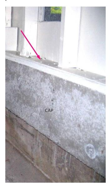
Another example: This is from the side. The red arrow point at where the end of the mudsill is supposed to be.
