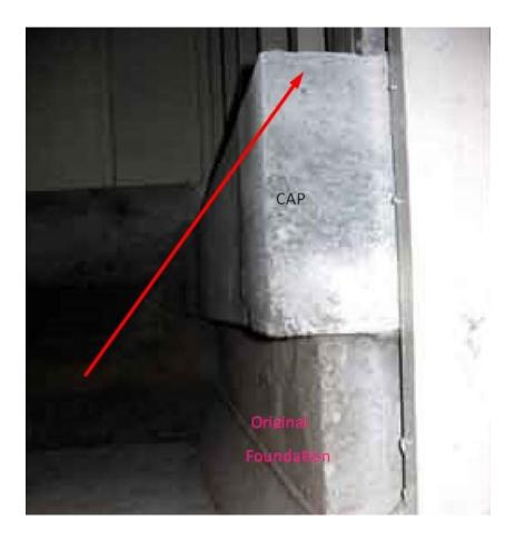
The concrete should have some reinforcing connecting the cap to the existing foundation but there is really no way to know.
