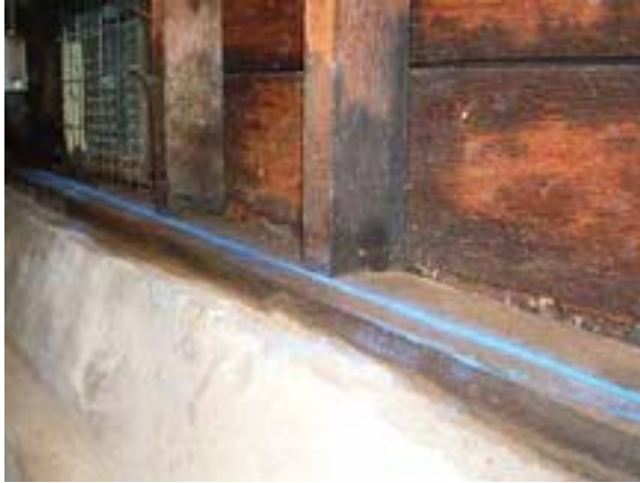
Illustration 3 Chalk line marks where the cut will be.
