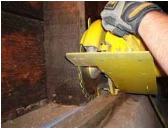
Illustration 5 Flush-cut saw cutting next to stud.
