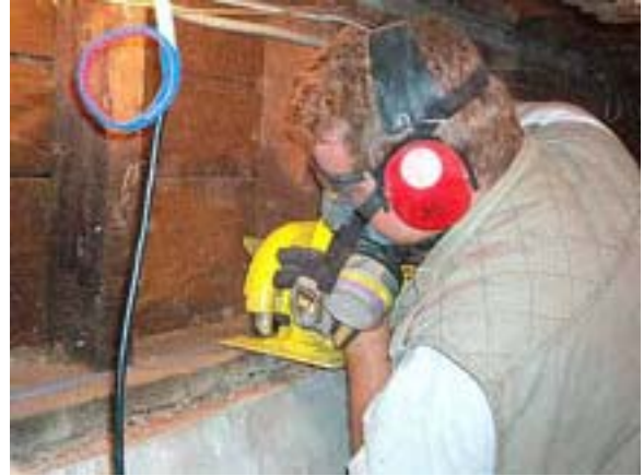
Illustration 4 Installer flush-cutting mudsill.
