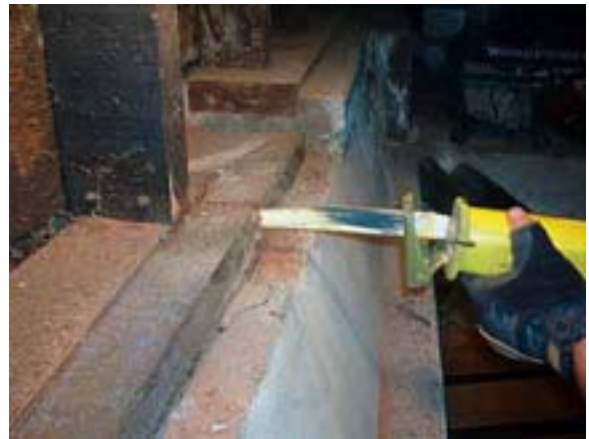
Illustration 6 Cutting the ends of the flush-cut sill.
