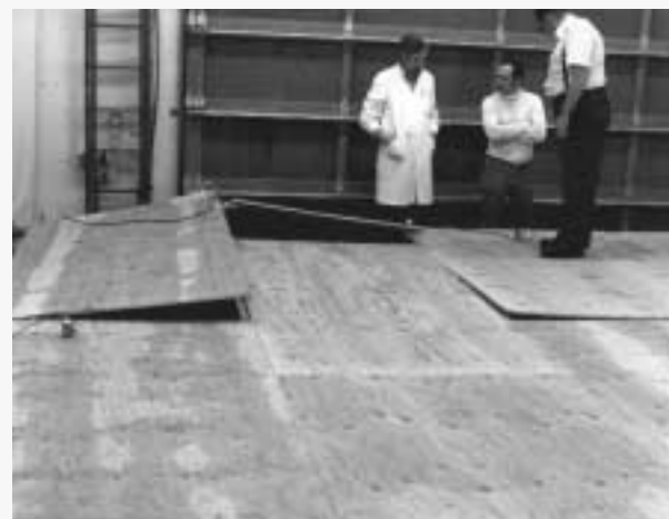
FIGURE 10 DIAPHRAGM 7 AFTER FAILURE.
