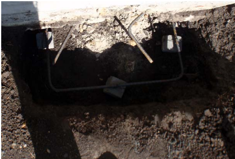
Image 13 All Rebar Installed.
