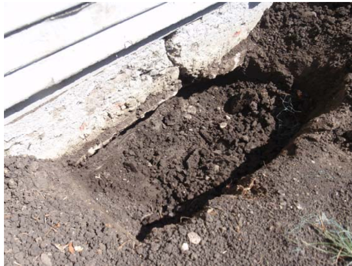
Image 11 Dig under crack for new concrete
