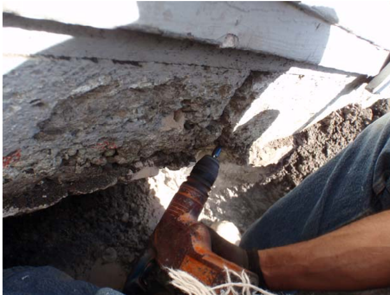
Image 12 Drilling into Foundation for Rebar
