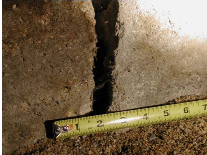
Image 10 Foundation Crack
