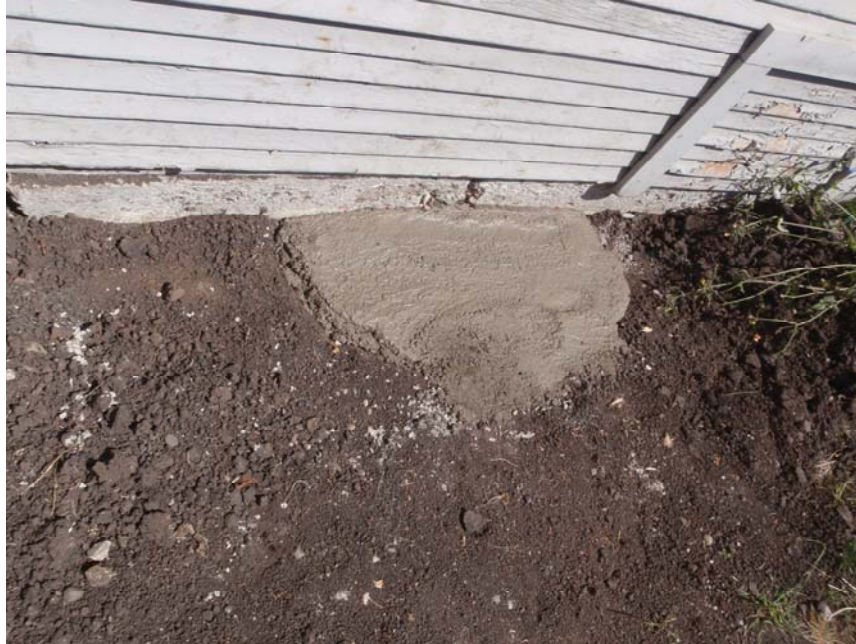
Image 14 Concrete in Hole
