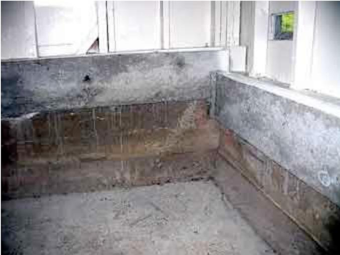
Foundations in the Bay Area are sometimes capped in order to increase the distance of the soil to the wooden walls. This is just as easily done with a shovel. In these cases it is important to use bolts that extend through the new foundation cap into the old foundation. This keeps the new foundation cap from sliding.
