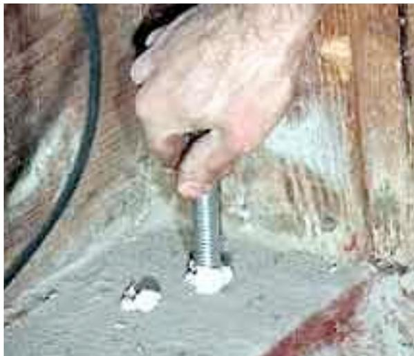
This is an installation of a hold down bolt being epoxied into the mudsill. It is important to make sure the hole is free of dust by brushing the hole out with the epoxy manufacturer's bottle brush and blowing the dust out with compressed air. Ideally the hole is blown out and brushed 3 times
