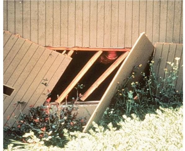
**Example 3:** Cripple wall failure from improperly installed plywood siding.
