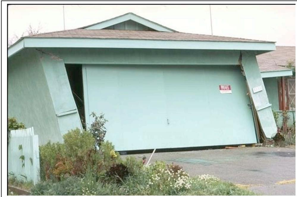
Overtuning damage caused to shear walls at front of garage.
