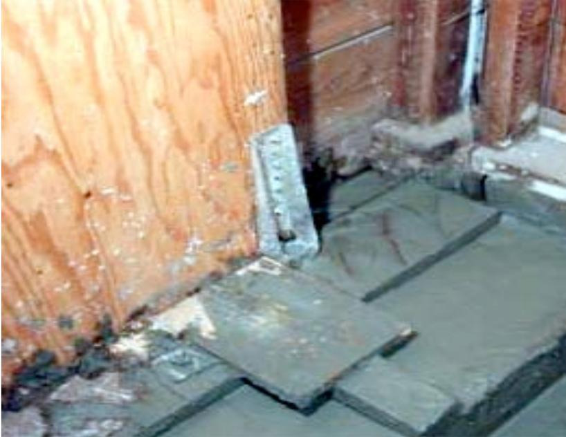
Here is the same view after the concrete has been poured and the plywood installed. An all-thread anchor rod with a nut at its lower end has been cast into each block of concrete to anchor the holdowns to the new concrete.
