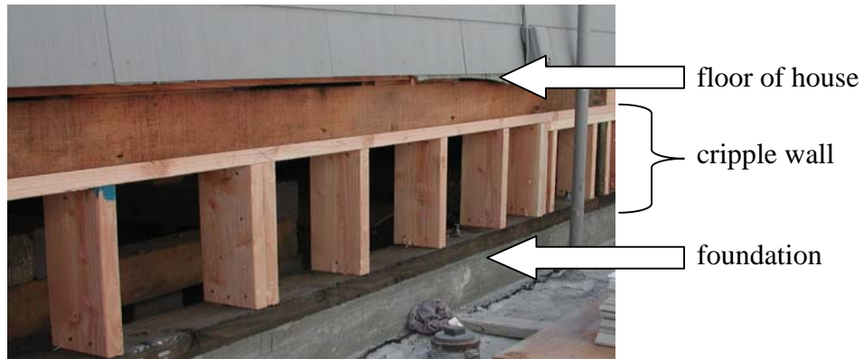
A typical cripple wall seen from the outside Photo courtesy Summerfield Inspections, Berkeley
