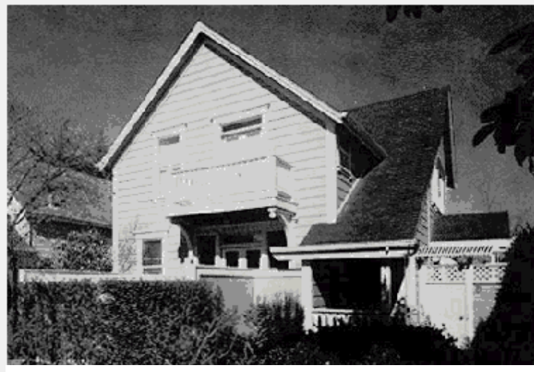
210 Elm Street in Santa Cruz saved by retrofitting
