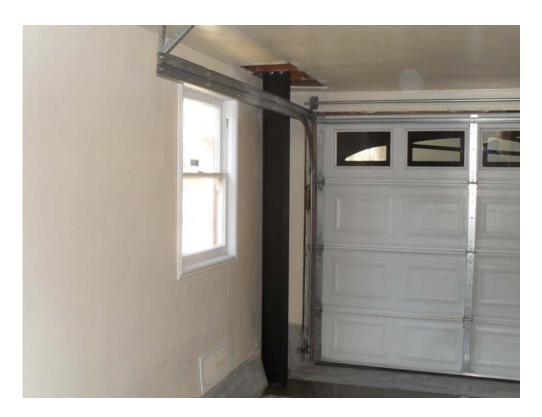
Embedding a very rigid large steel beam (the black upright column to the left) into concrete and attaching it to the floor above the garage door opening addresses this weakness. These are known as cantilevered columns.
