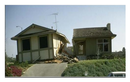
Again, by way of illustration of a simple engineering concept, the narrow walls on either side of the garage can tip over.
